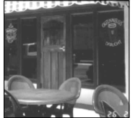
Rehabilitated storefront with incompatible stained glass door.
