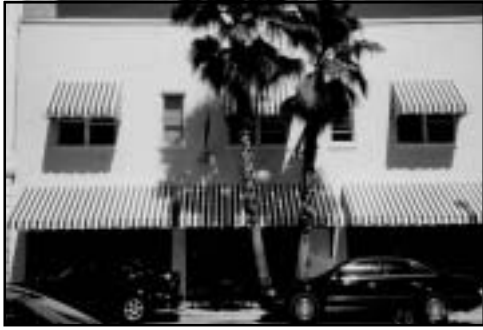
Rehabilitated 1920s commercial building.
