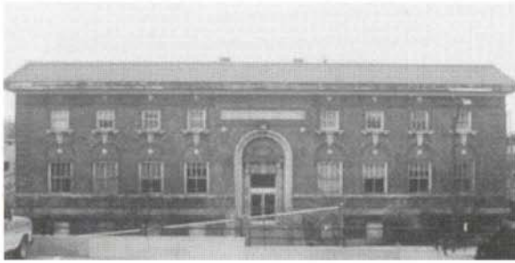
The Sioux City Free Public Library prior to rehabilitation. The building had major structural problems after sitting vacant for over ten years.
