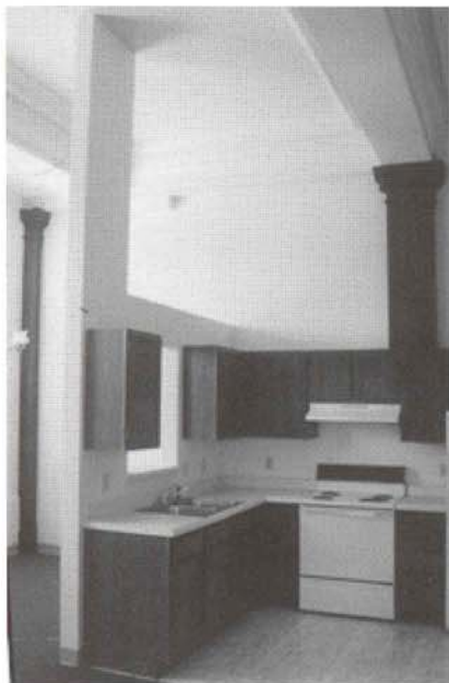
The historic beamed ceilings and trim remain visible by constructing low dividing walls approximately six feet below original ceiling heights, and by not lowering the ceilings in primary spaces.
