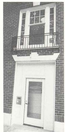
Code issues were met with creative solutions. Accessibility is provided by modifying an original window into a doorway. The balconets were retained by adding a hidden hinge allowing egress.
