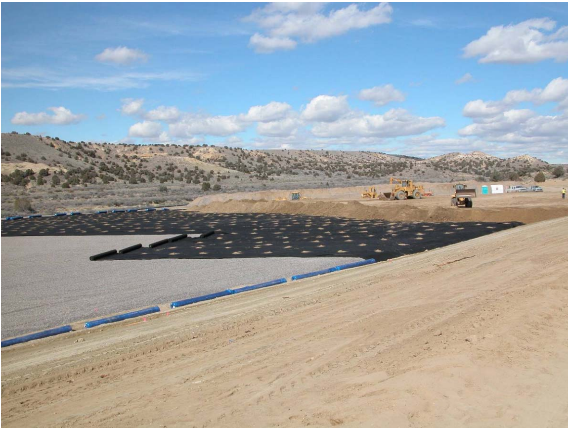
Figure D-1.0-5. Capillary barrier under construction on Superfund site, Farmington, NM
