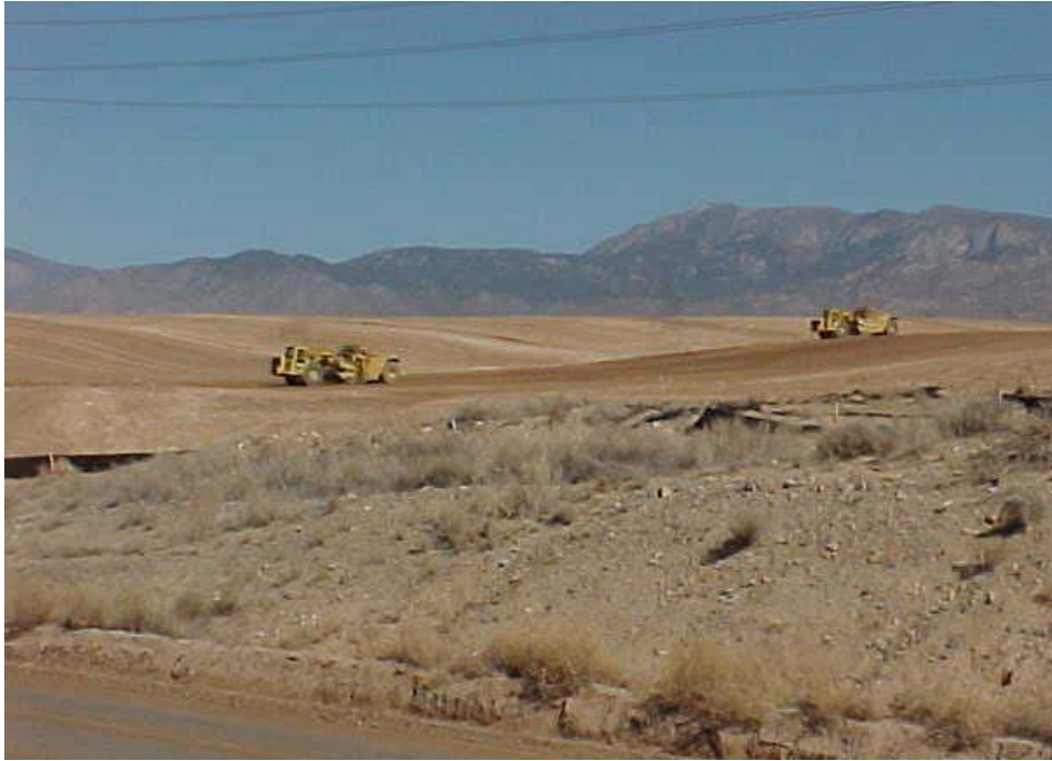
Figure B-2.2-1. ET cover installation on Kirtland Air Force Base
