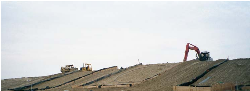
Figure B-2.1-2. Finley Buttes Regional Landfill test covers installation
