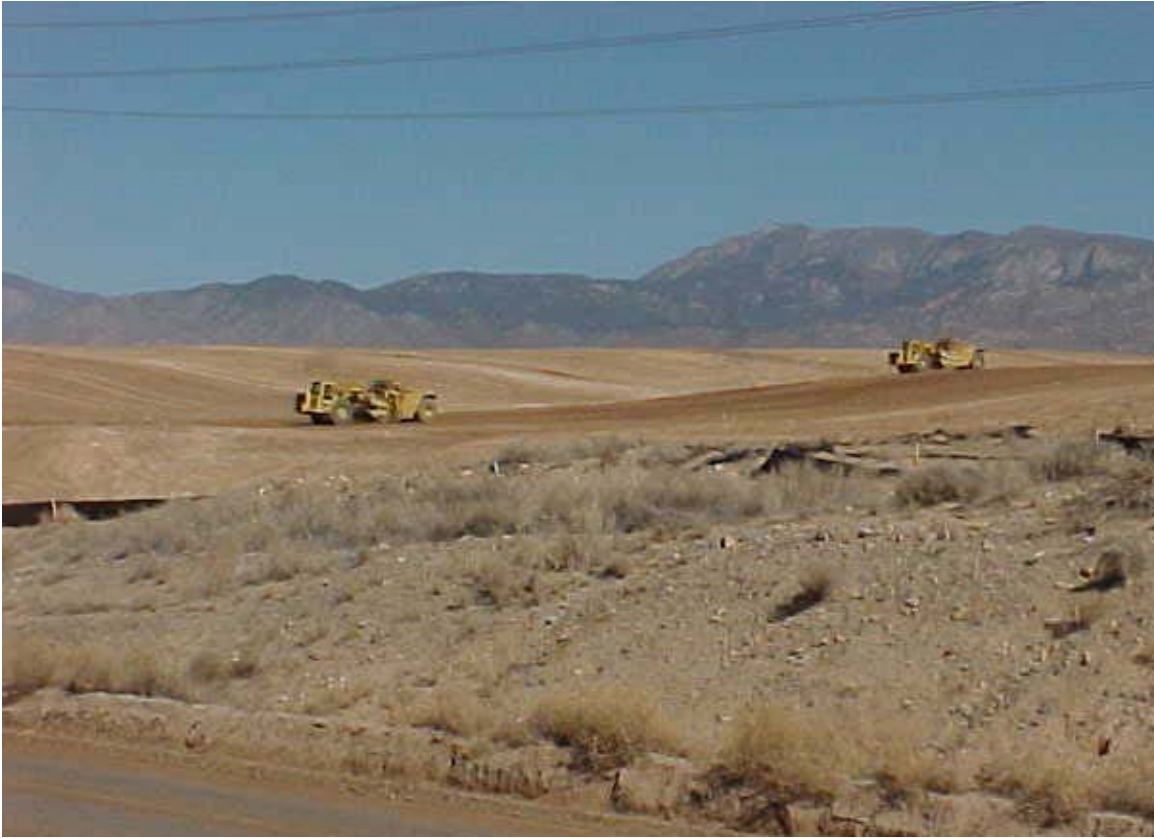
Figure 2.2-4. ET cover under construction on Kirtland Air Force Base, Albuquerque, NM
