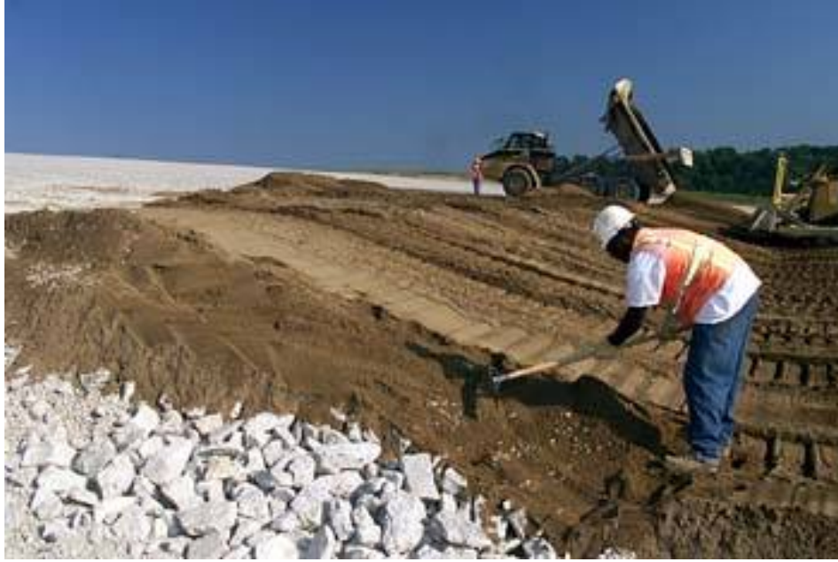
Figure 4-2.3. Installing cobble bio-barrier in cover system at Fernald, Ohio
