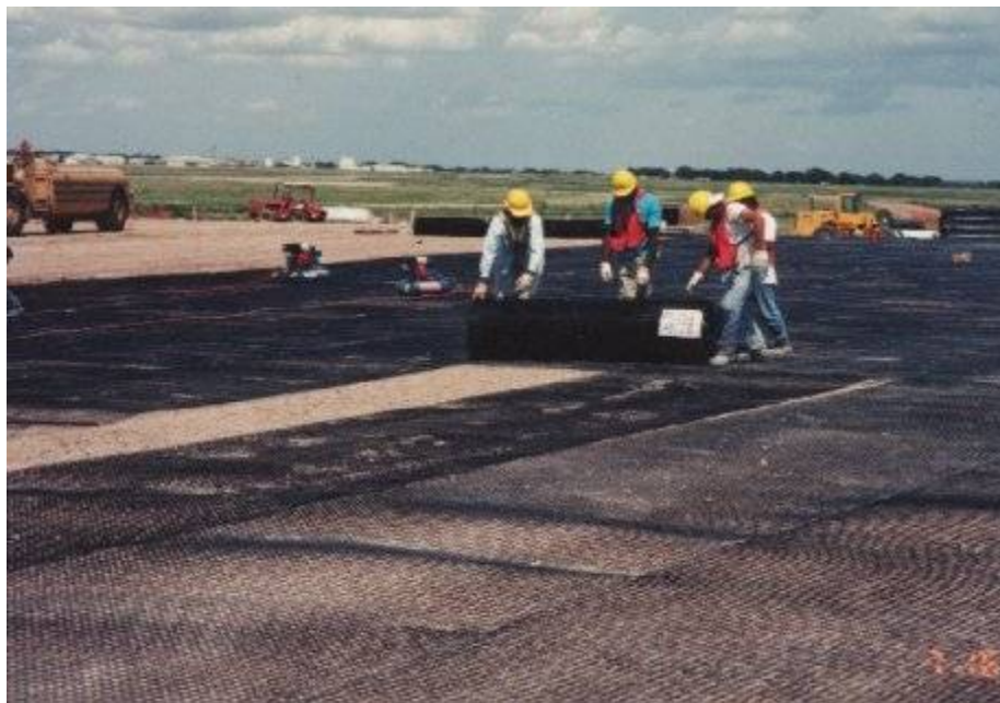
Figure 4.2-7. Placing wire mesh bioinvasion layer
