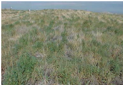
Figure 4.1-3. ET cover – 3.5-ft-thick soil layer
