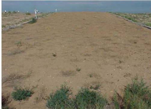
Figure 4.1-2. Multilayered cover with a thin (1-ft-thick) top soil layer
