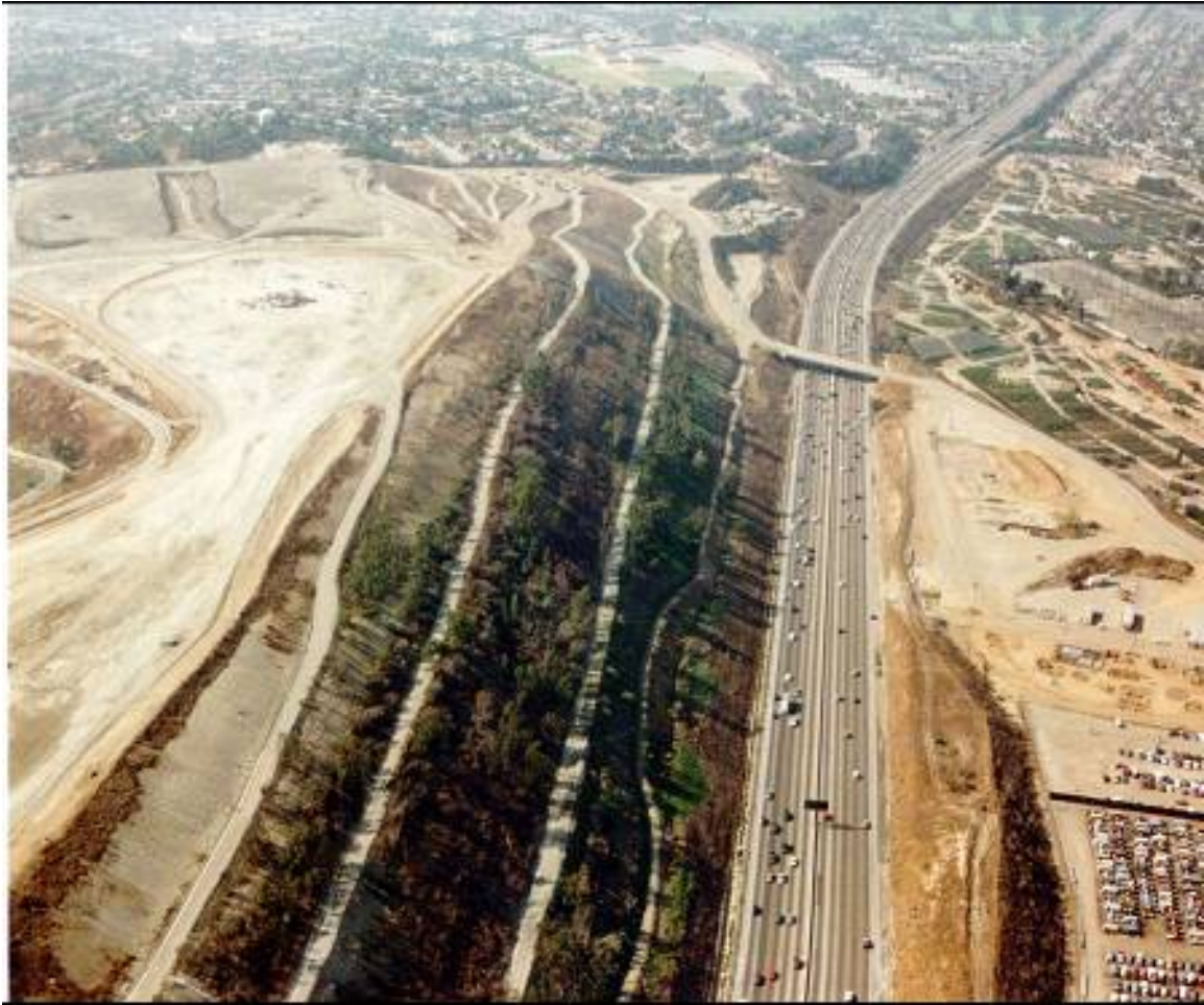
Figure 2.2-5. Oil Landfill: ET cover in southern California
