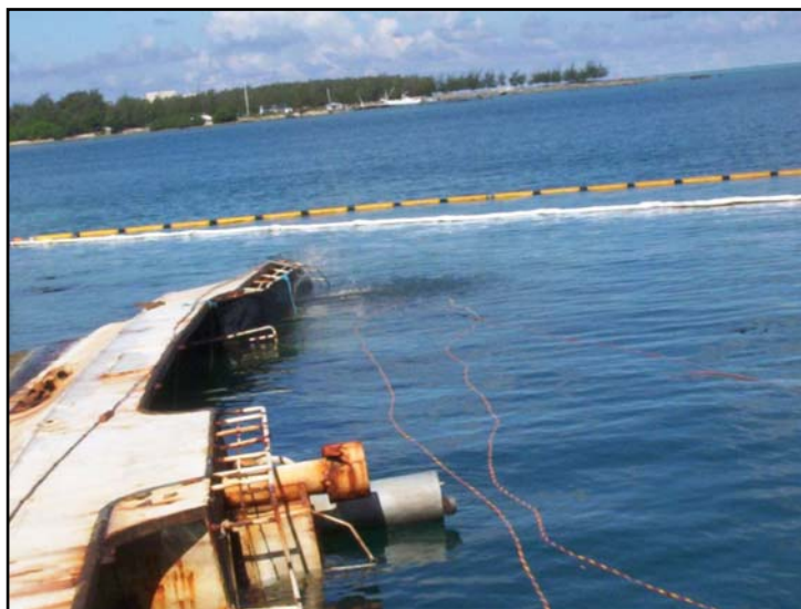
Grounded vessel being cut underwater (black water)
