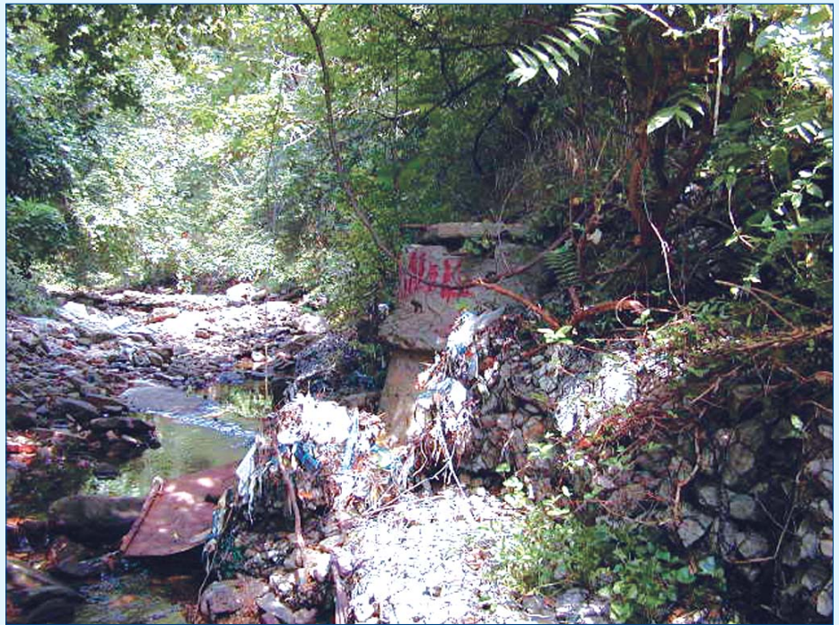
An urban stream impacted by wastewater leaking from deteriorating sewer lines at Maidens Choice Run upstream from USGS stream-gaging station 0158935, Baltimore, Maryland. [Photo by Gary T. Fisher, U.S. Geological Survey]
