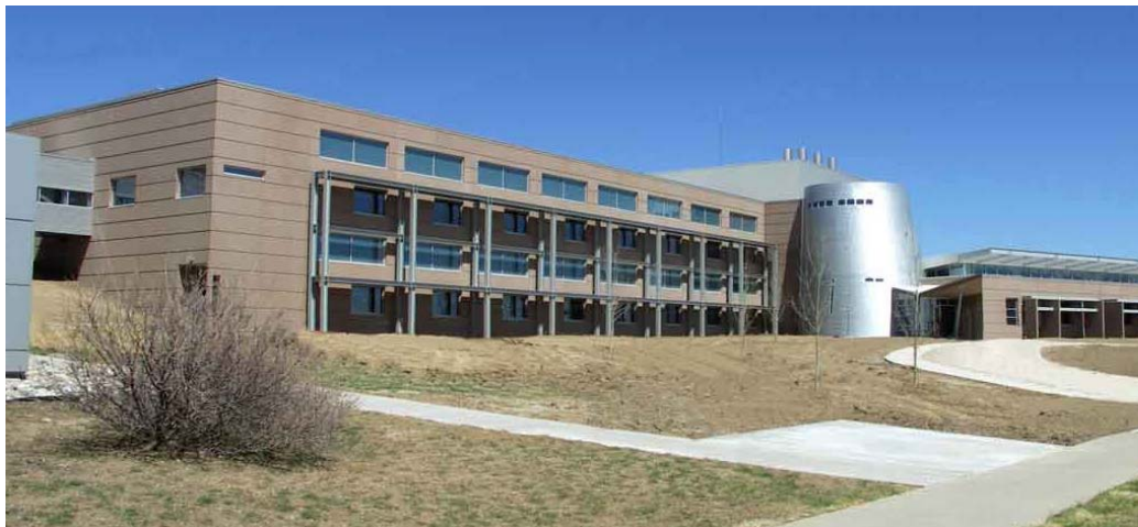
Construction of NREL's Science and Technology Facility is expected to be substantially complete in May.
