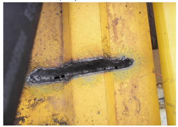
If crack has propagated through the thickness of the top plate; open up enough of a groove to allow for inserting a backing plate made of A36 material. This is recommended to ensure complete joint strength.
