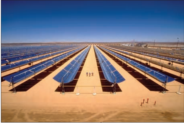
Solar power facility at Kramer Junction, California.
