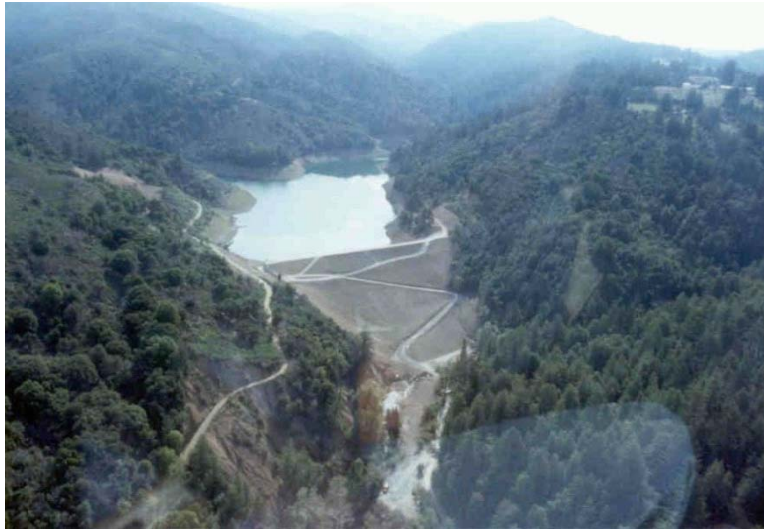
Fig. 2-7 Aerial view of Austrian Dam (Photograph: Courtesy of David Gutierrez)
