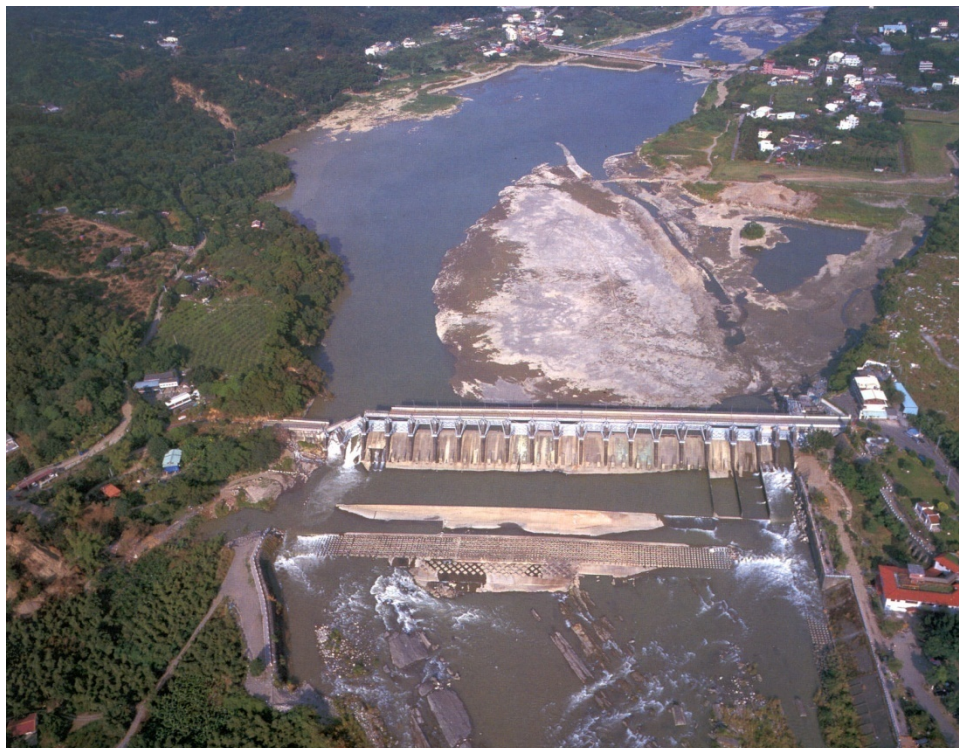
Fig. 2-5 View of dam after the 1999 Chi-Chi Earthquake showing damage to portion of dam due to fault rupture
