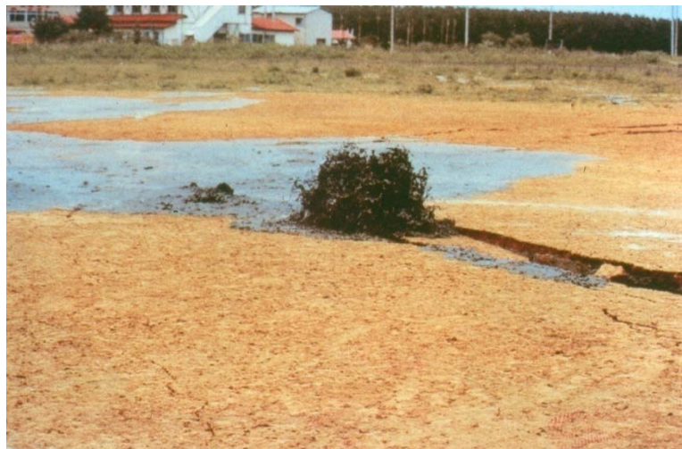
Fig. 2-11 Surface evidence of liquefaction triggered during the 1978 Miyagi-Ken-Oki earthquake in Japan
