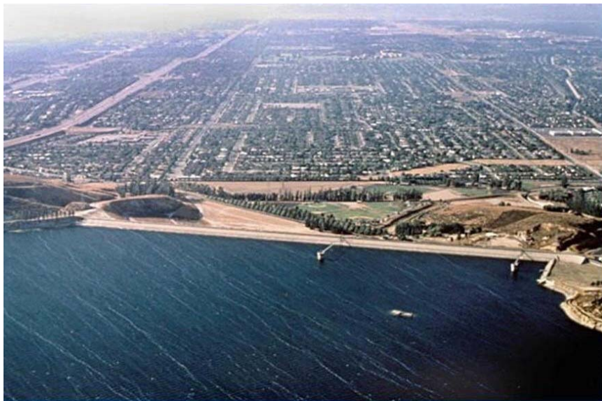
Fig. 2-15 Aerial view Lower San Fernando Dam before the occurrence of the 1971 San Fernando Earthquake showing the extensive number of residences that would have been affected by a breach of the dam (Photograph: Courtesy of David Gutierrez)
