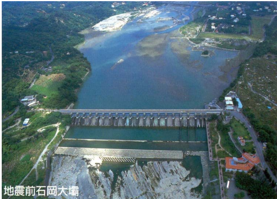
Fig. 2-4 View of dam in Taiwan prior to the occurrence of the 1999 Chi-Chi earthquake
