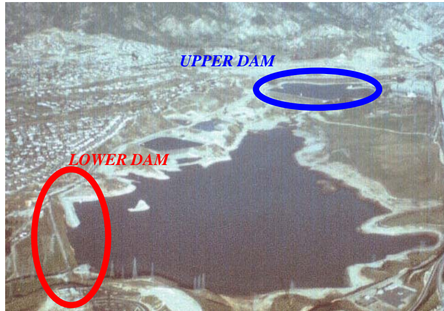
Fig. 2-12 San Fernando Dam Complex shortly after the occurrence of the 1971 San Fernando earthquake
