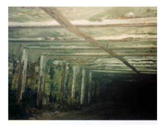
Another dangerous situation can occur if the posts that are supporting beams become dislodged, such as being struck by a haulage vehicle.
