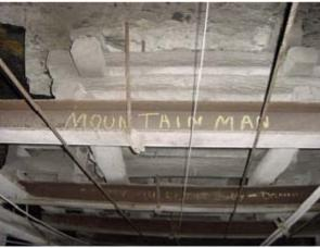
By adding these types of supports, the roof beams themselves will not create a falling-material hazard if the posts (or coal ribs) supporting them are inadvertently dislodged.
