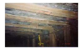
Collapse of roof beams can be prevented in these situations by running straps or suspended cable supports under the beams, or by bolting the beams.
