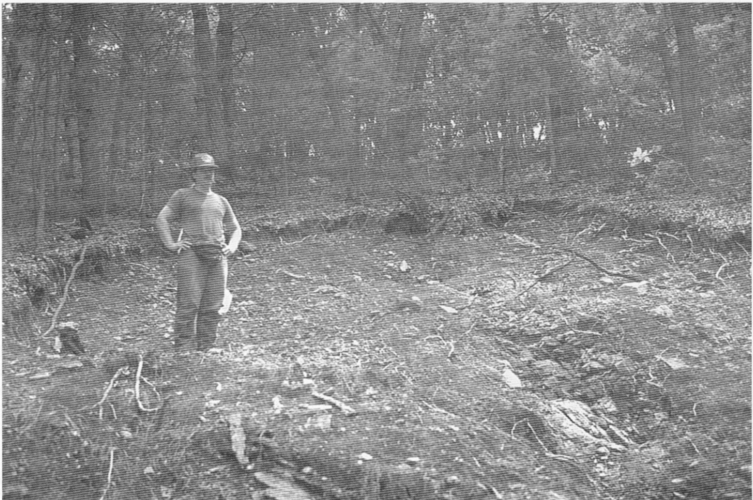
Figure 7. Shallow planar slide in colluvium over weathered granitic bedrock, scarp about 0.7 m deep and about 9 m wide near Camp Shiloh.
