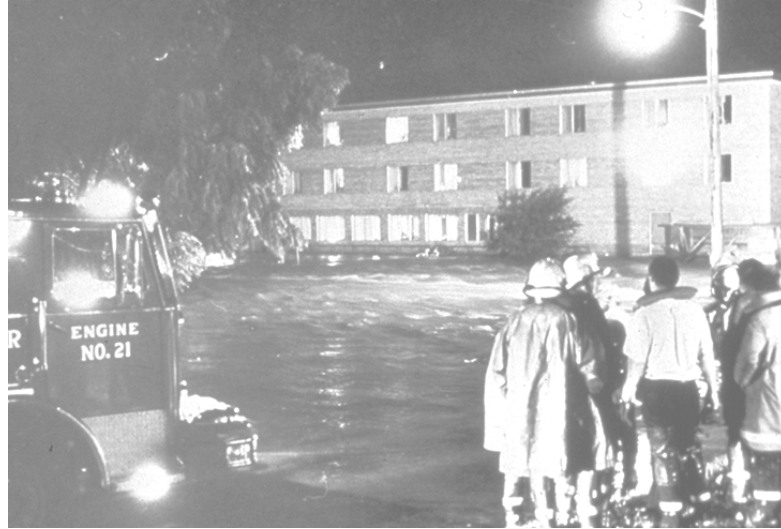
Figure 6-4: Four people died in a 1978 flood in this critical facility. This nursing home in Rochester, Minnesota, was isolated by high velocity floodwaters. Because there was no dry land access, firefighters could not rescue the occupants.
