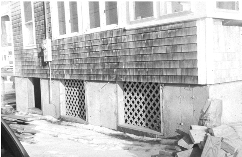
Figure 5-10: Building elevated on crawlspace with openings.
