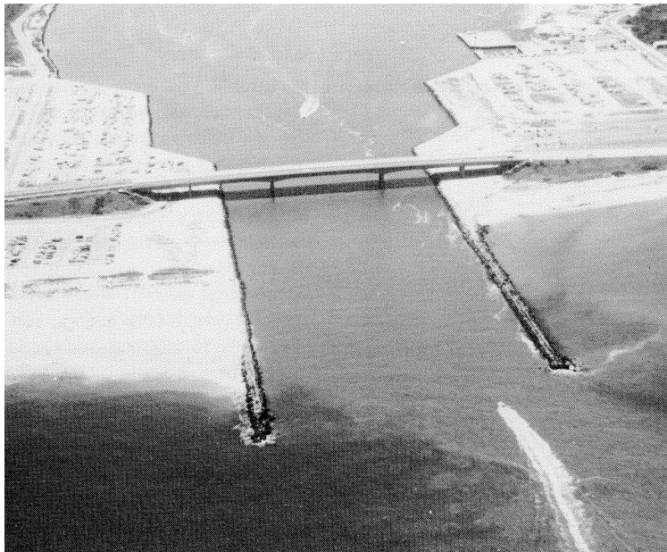
Figure 1-14. Jetties to protect a navigation inlet affect sand accumulation and erosion.
