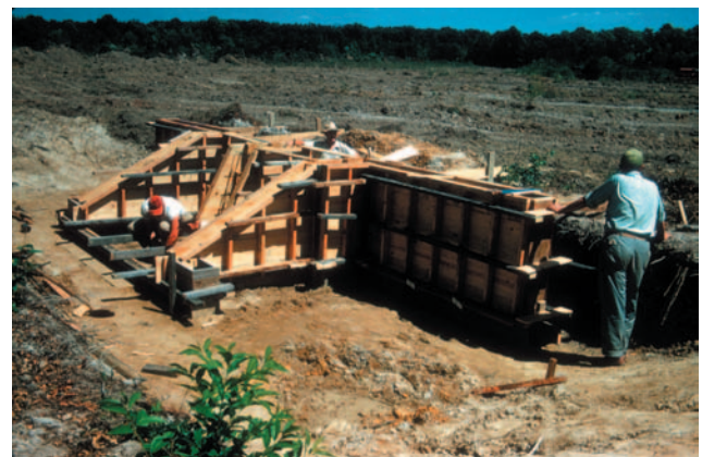
Construction of a water control structure for an impoundment in 1954
