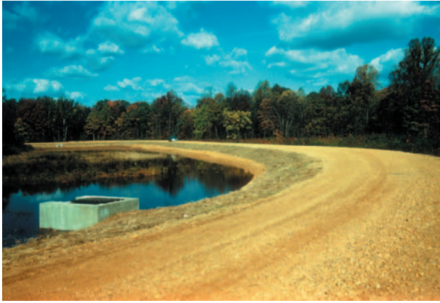
Completed impoundment showing water control structure
