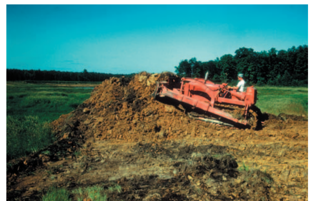
Creating an island in an impoundment basin
