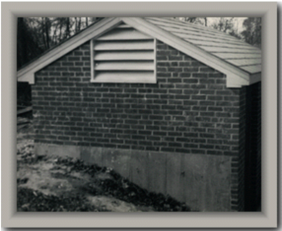
Pump house for spring reservoir
