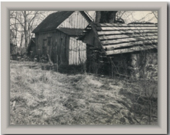
Ice storage and poultry house on site of Nelson Laboratory
