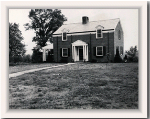
Superintendent's residence constructed with WPA-PWA grant
