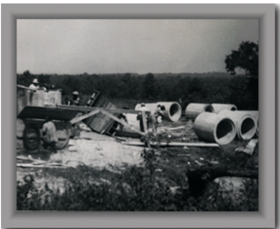
Construction of large concrete pipe by refuge WPA workers
