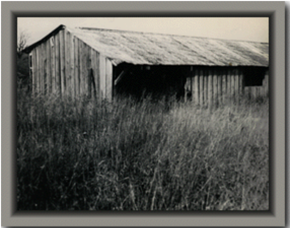
Shed for cattle and sheep razed in connection with the construction program
