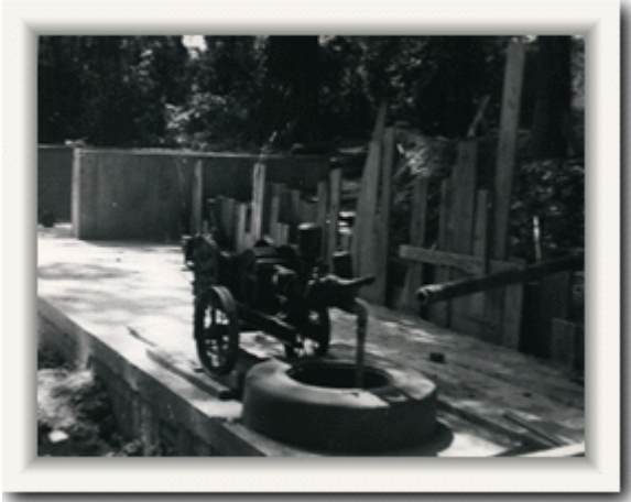
Construction of 20,000 gallon reservoir for storage of spring water
