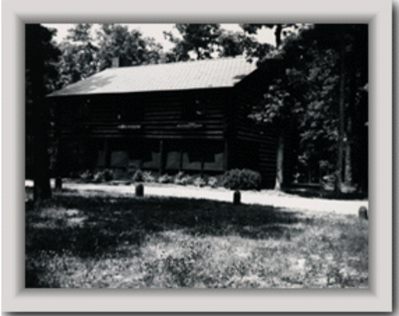
Log house following repair and landscaping work
