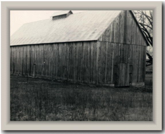
One of two large tobacco barns rebuilt as storage warehouses by WPA
