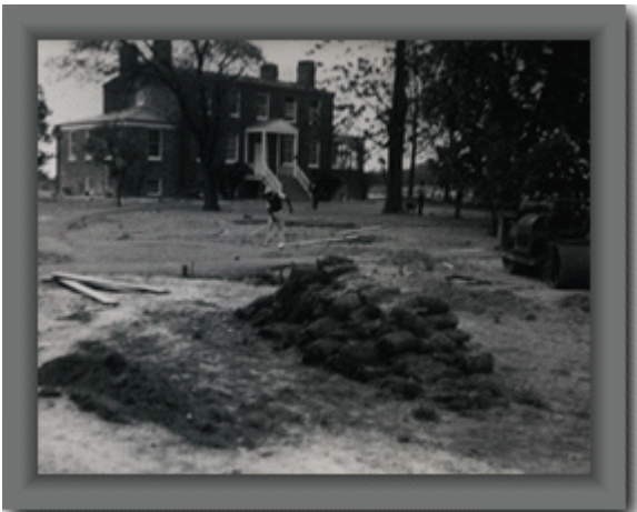
Sidewalk construction, grading, and sodding prior to dedication day
