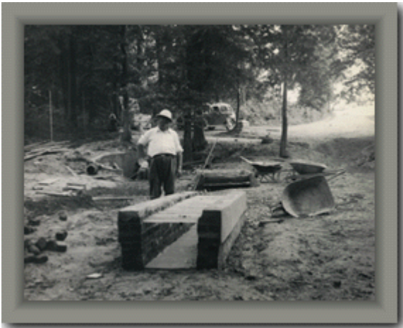
Constructing barbecue pit and spring reservoir for headquarters picnic ground
