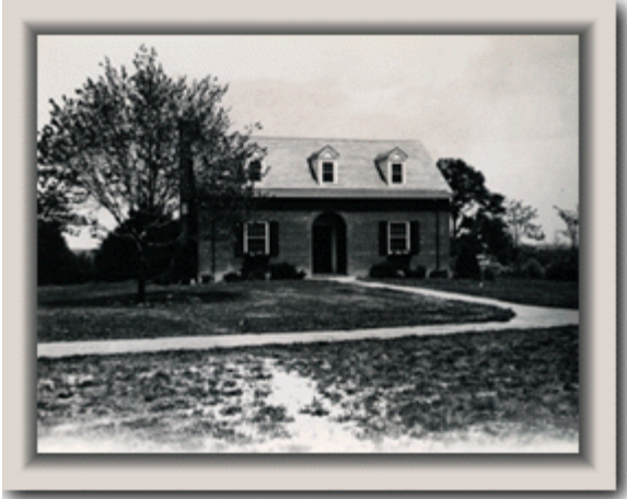
Assistant Superintendent's residence
