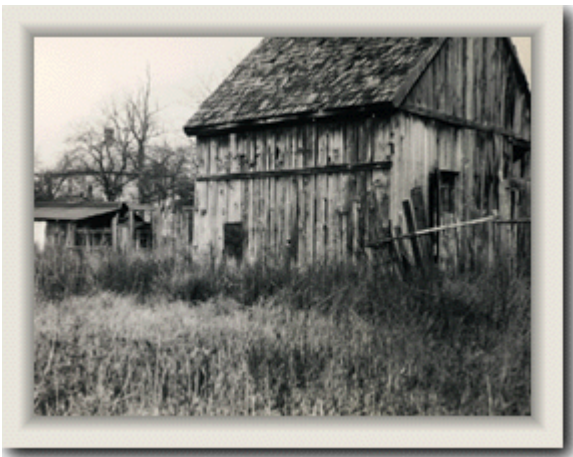
Barn and outbuildings on Harding farm razed to provide for new construction
