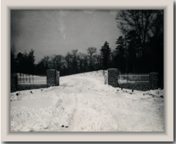
Entrance gates and road to refuge headquarters
