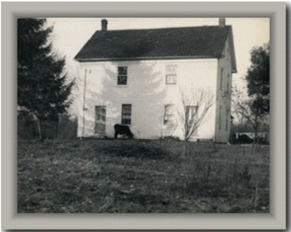
Residence on J.W. Knowles farm razed in connection with new construction described in Fiscal Year 1945
