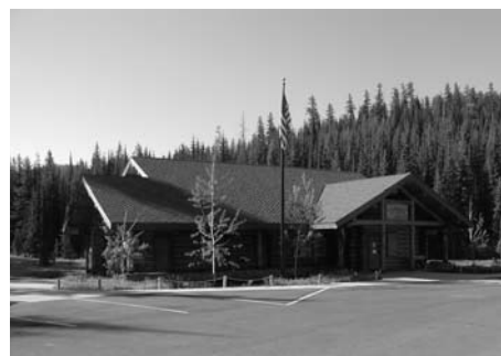
The new Lolo Pass Visitor and Rest Area. Located at 5,225 feet on the border between Idaho and Montana, the new structure includes restrooms, exhibits, an interpretive trail, a sales area, and a warming hut for winter recreationalists.
