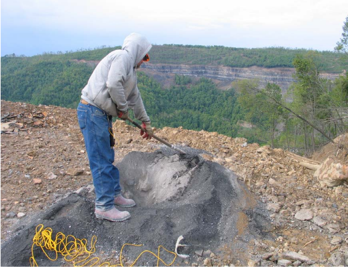
Figure 14 - Stemming a blasthole
