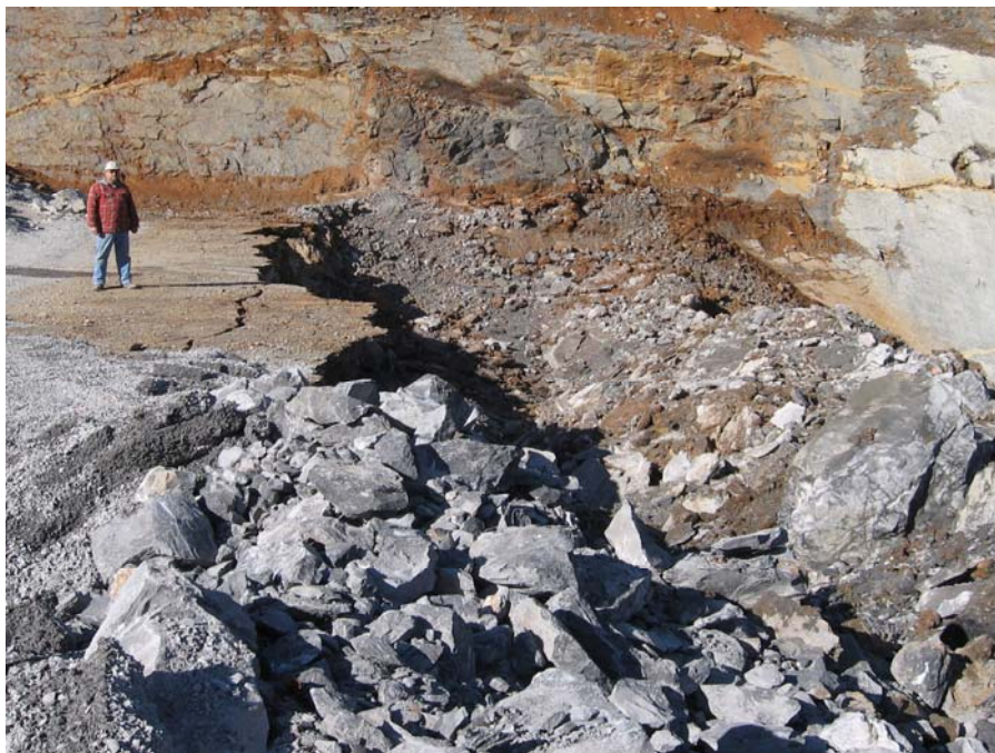
Figure 11 - Muck pile of the blasted material
