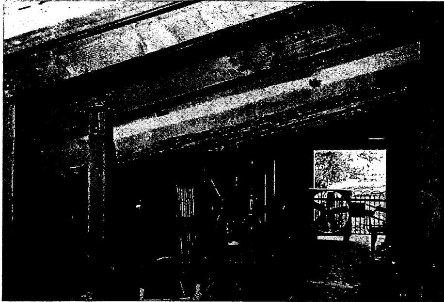
Figure 1: View of interior space below east bleacher, looking east to exit. Note exposed reinforcing bars and shoring due to failing concrete structure. Photo dated March 2005 by ARG.
