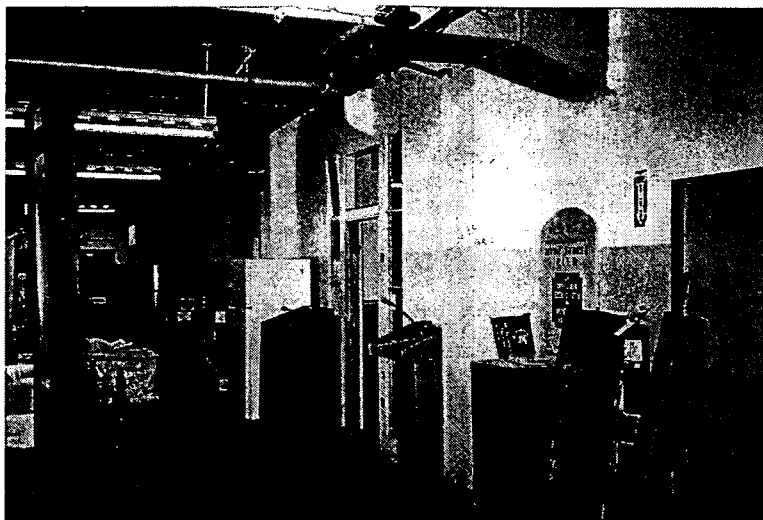
Figure 14: View of passage below central bleacher, looking east. Photo dated March 2005 by ARG.
