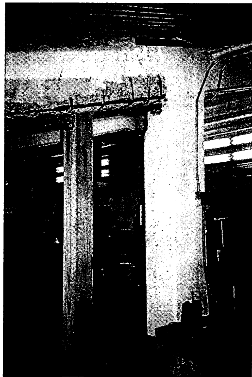
Figure 2: Detail view of exposed reinforcing bars and concrete spalling in interior space below east bleacher. Photo dated March 2005 by ARG.
