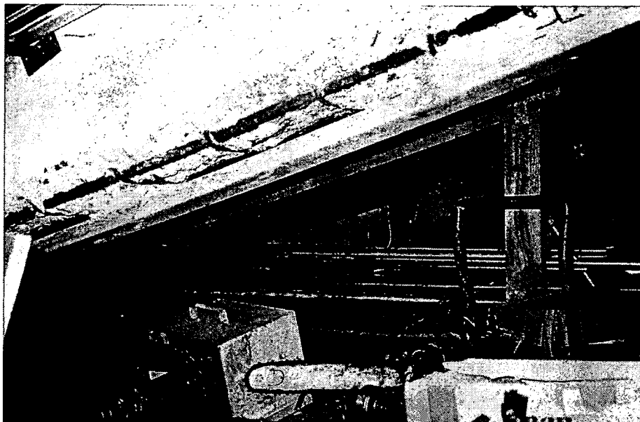
Figure 3: Detail of spalled concrete below east bleacher. Photo dated March 2005 by ARG.
