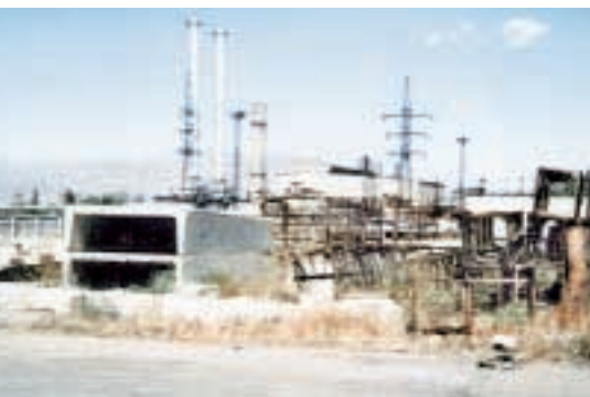
Uranium facility at Chkalovsk, precious metal upgrading facility and pumping station.
