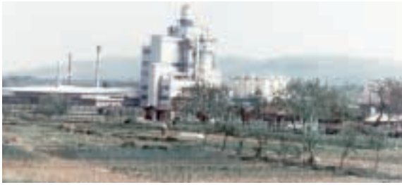
Merima Chemical Plant. Krusevac, Serbia
