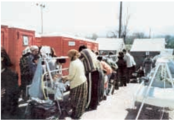
Chemical toilets and basins in Kosovar refugee camp set up by German unit in Macedonia.
