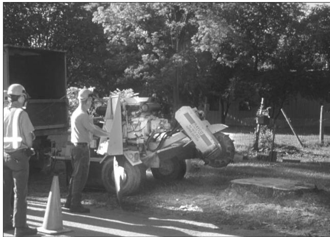
Using a grinder to remove tree stumps causes minimal site disturbance and allows replanting in the same location.
