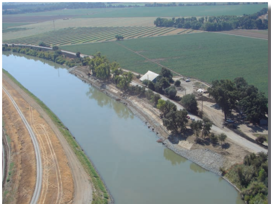
Levee repairs in California's Central Valley (photo courtesy of California DWR)
