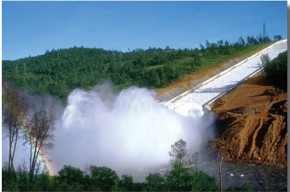
Oroville Dam spillway (photo courtesy of California DWR)
