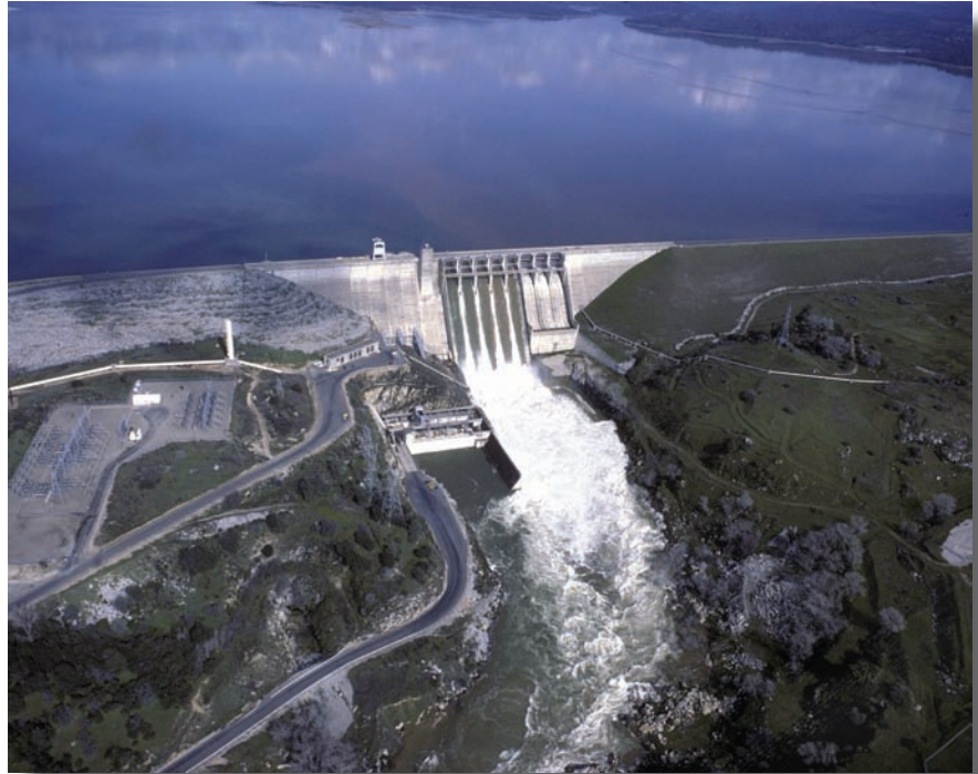
Folsom Dam (photo courtesy of USBR)
