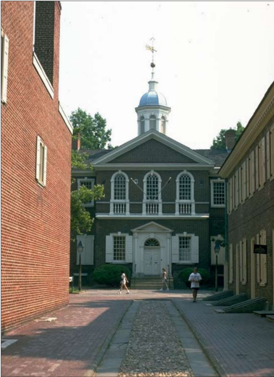
The Carpenters' Company of Philadelphia, the oldest trade guild in America, has owned Carpenters' Hall since 1770. The first Continental Congress met here in 1774.
