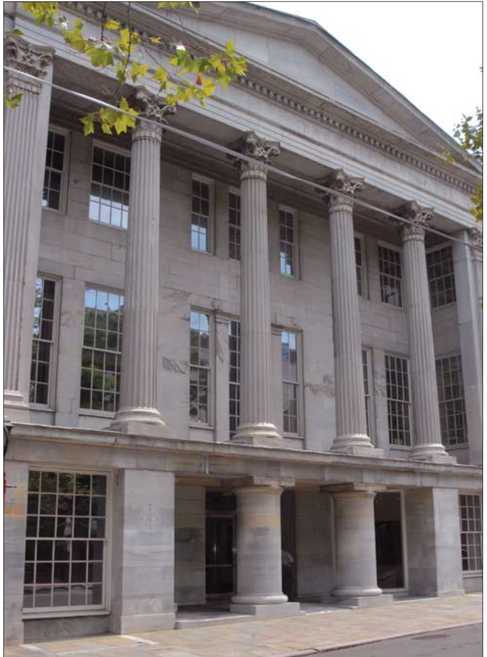
The Merchants Exchange Building has been adaptively restored and is the home of the park's library, training room and administrative offices.
