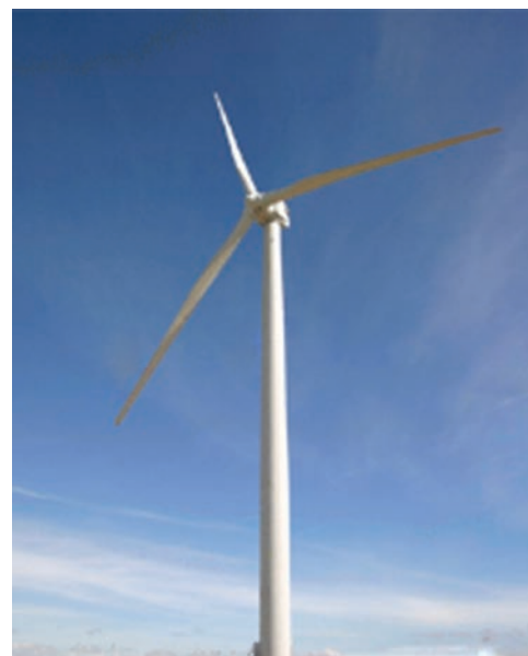
Clipper 2.5-MW Liberty Turbine installed in Medicine, Wyoming.
