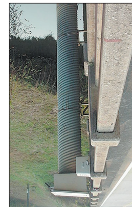
Typical flood-monitoring gage well and a gage house that is composed of a water stilling well. Gages are normally mounted to bridges and river stage data are transmitted to the USGS Georgia Water Science Center in Atlanta.
