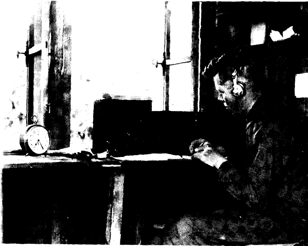
Interior Intercept Station #1, Verdun
