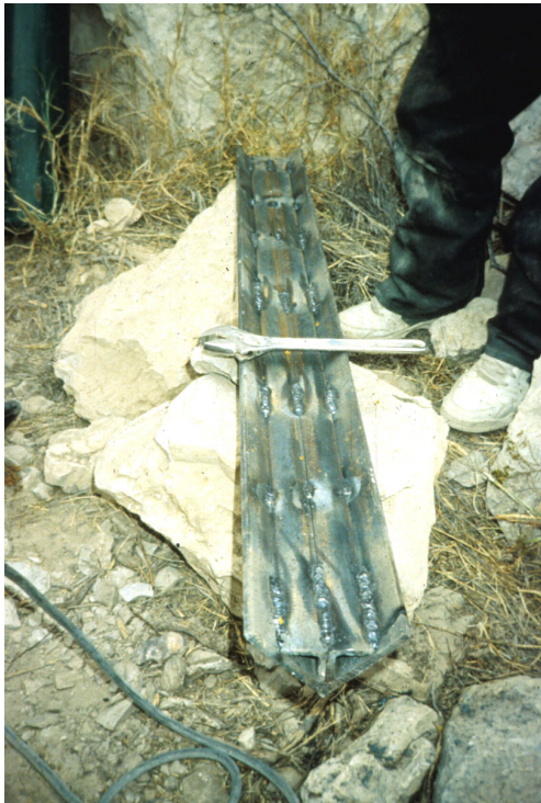
Bat gate fabrication at Big Bend National Park (ACCA design). Notice 1"-diameter steel pin anchors to sill and ribs, L4"x4"x \frac{3}{8} " angle steel for structural members and cross member supports with two L1 \frac{1}{2} "x1 \frac{1}{2} "x \frac{1}{4} " angle steel "stiffeners" welded inside each horizontal cross member, and grinding of all rough edges to avoid sharp spots that would otherwise injure bats.
