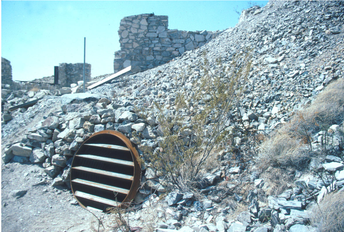
Figures 3 and 4. Culvert-mounted bat gate installed to preserve unstable mine entrance, and bat cupola installed on shaft, Mariscal Mercury Mine, Big Bend National Park, Texas. (1995)
