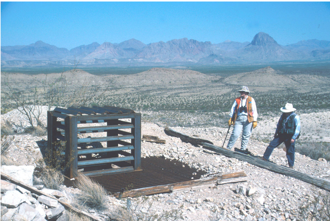
Figures 3 and 4. Culvert-mounted bat gate installed to preserve unstable mine entrance, and bat cupola installed on shaft, Mariscal Mercury Mine, Big Bend National Park, Texas. (1995)
