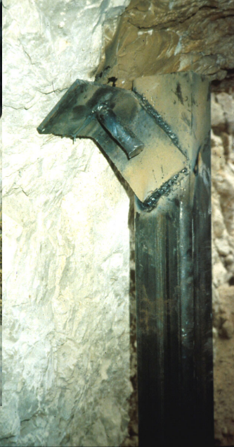
Bat gate fabrication at Big Bend National Park (ACCA design). Notice 1"-diameter steel pin anchors to sill and ribs, L4"x4"x \frac{3}{8} " angle steel for structural members and cross member supports with two L1 \frac{1}{2} "x1 \frac{1}{2} "x \frac{1}{4} " angle steel "stiffeners" welded inside each horizontal cross member, and grinding of all rough edges to avoid sharp spots that would otherwise injure bats.
