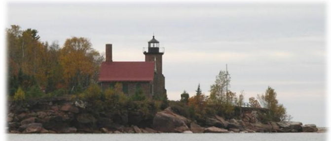
Sand Island Lighthouse, Apostle Islands, Lake Superior; photo courtesy Jay Glase, NPS
