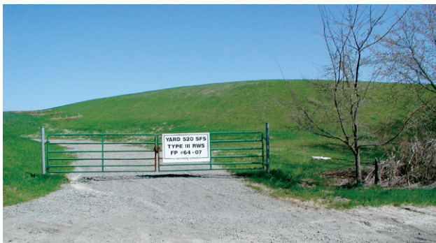
Yard 520 Fly Ash Landfill. Water table mounding beneath landfills can be subtle, but the effect on shallow ground water flow can have serious consequences. (Scott Hicks, INDU)
