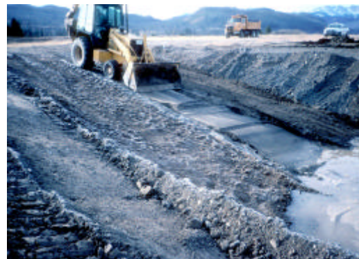
A park equipment operator places parallel strips of mine reject material, sand, and topsoil in preparation for willow establishment experiments. These experiments identified the combination of soil type and water table elevation that would optimize willow establishment from seed.
