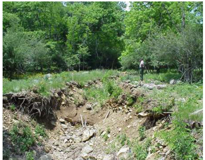
Lower headcut prior to stabilization, looking upstream. Note raw vertical banks, exposed soil, and small amount of groundwater drainage at the face of the headcut.
