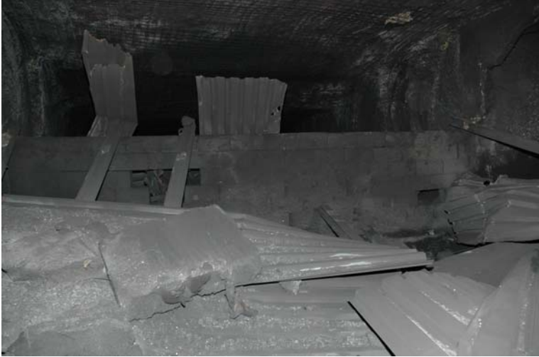
Figure 7 - Damaged Overcast at 58 Crosscut, No. 4 Belt
