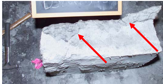
Figure 19 - Mortar in Vertical Joint
