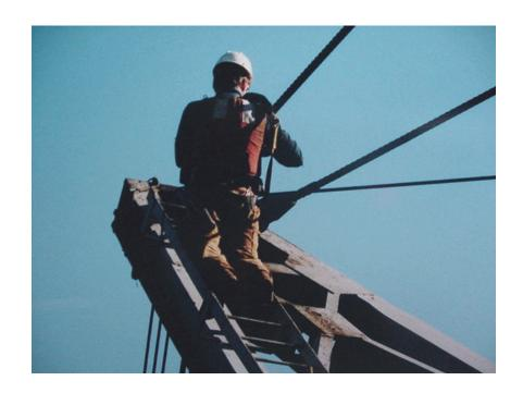
This module describes basic job steps, potential hazards and accidents, and recommended safe job procedures for <u>inspecting and replacing wire ropes</u>. The term "wire rope" is used in this module, rather than "cable," to avoid any possible confusion with electrical cables. This module is not intended to cover wire ropes that are used for hoisting persons.
