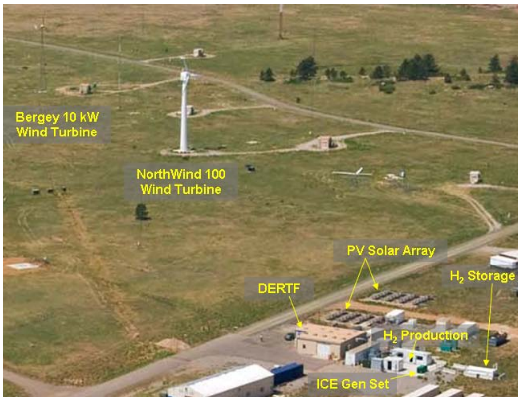
Figure 2-1: Aerial photograph of Wind2H2 site and equipment
