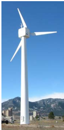
Figure 2-17: 100 kW NorthWind 100 turbine located at NREL's NWTC
