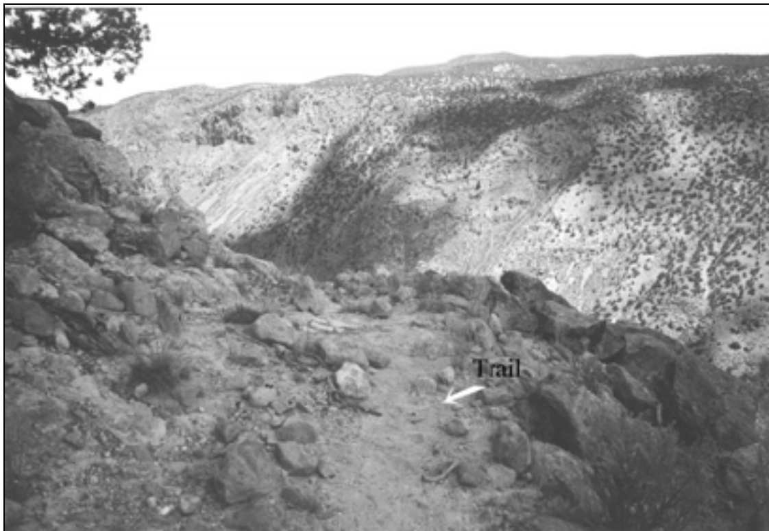
Figure 81.1. LA 134901 as it descends from the Portero del Rito into White Rock Canyon, illustrating cleared talus trail construction.
