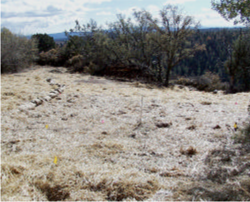
Straw and sandbags to control runoff at Solid Waste Management Unit 21-014
