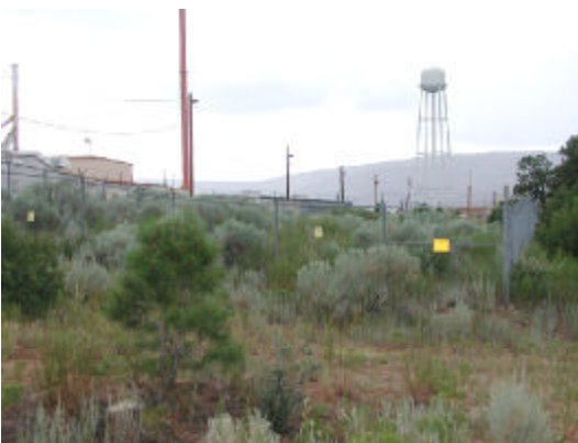
Material Disposal Area U
