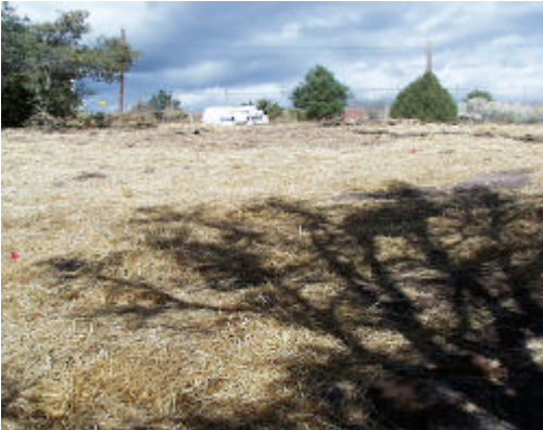
Straw in place to control runoff at Solid Waste Management Unit 21-014
