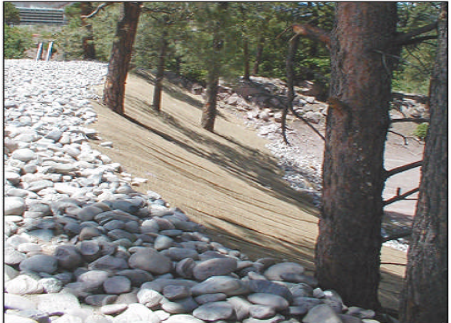
Potential Release Site 03-056(c) after cleanup activities
