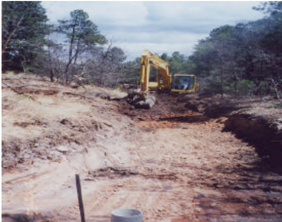
Excavation of contaminated soil
