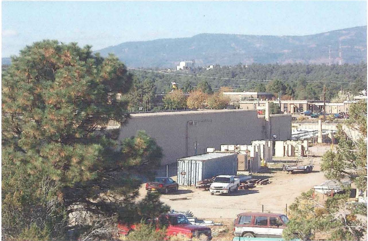
TA-53-3 Sectors A and B North side of building
