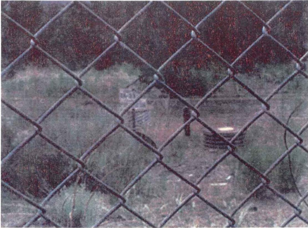
TA-33-93 Sanitary Sewer Septic Tank
