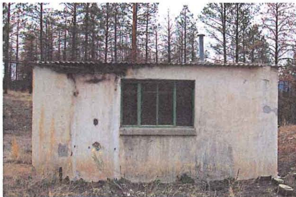
Photo 1c. View of east side
