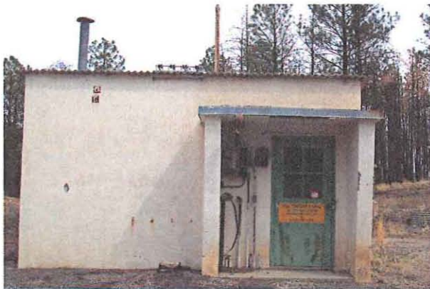
Photo 1a. View of west side
