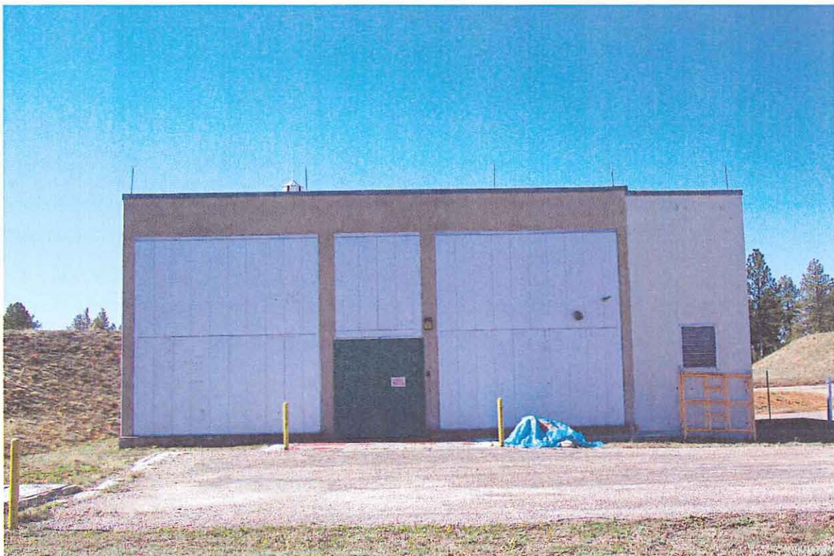
TA-9-35, north side
