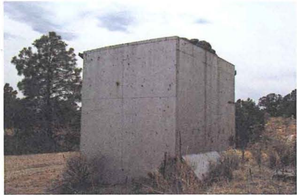
Photo 5b. Oblique view of east and north sides of TA-15-138
