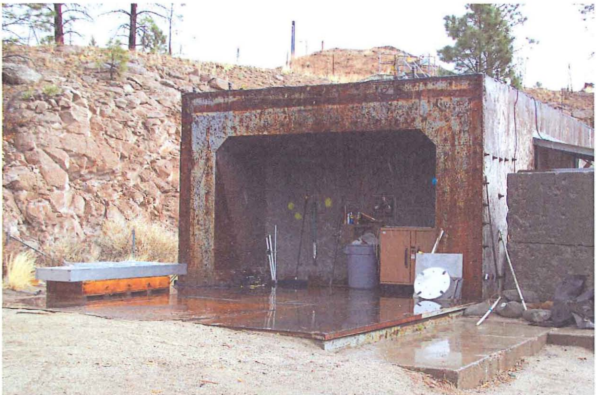
TA-40-4, southwest side
