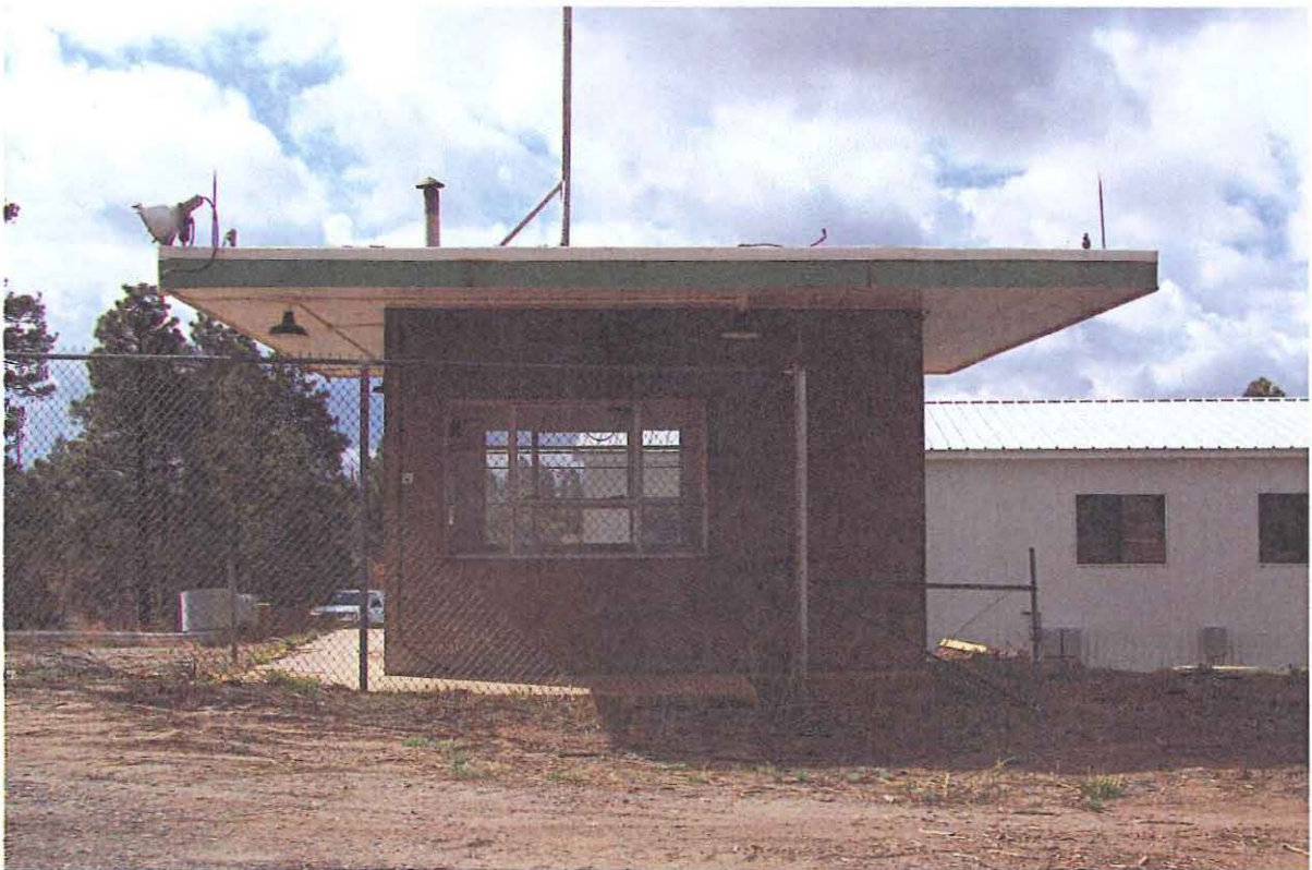
TA-40-19, north side
