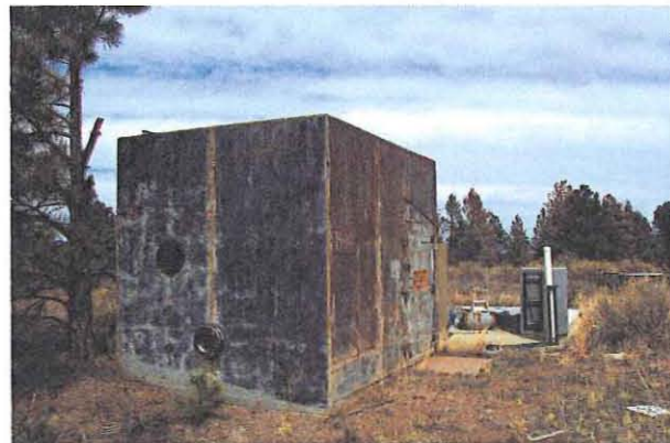
Photo 5d. Oblique view of west and south sides of TA-15-141
