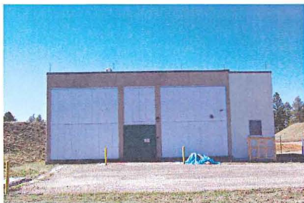
Photo 1c. View of north side of TA-9-35
