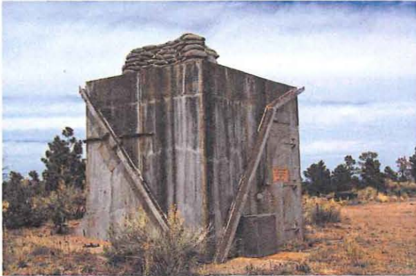
Photo 5a. Oblique view of west and south sides of TA-15-138
