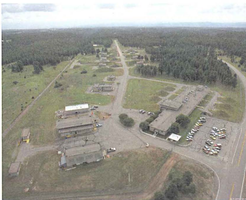
Figure 1. 1991 Aerial of TA-9
