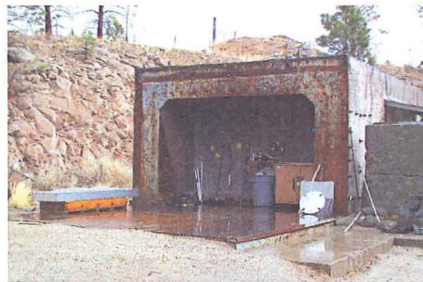
Photo 6b. Southwest end of structure showing firing chamber of TA-40-4
