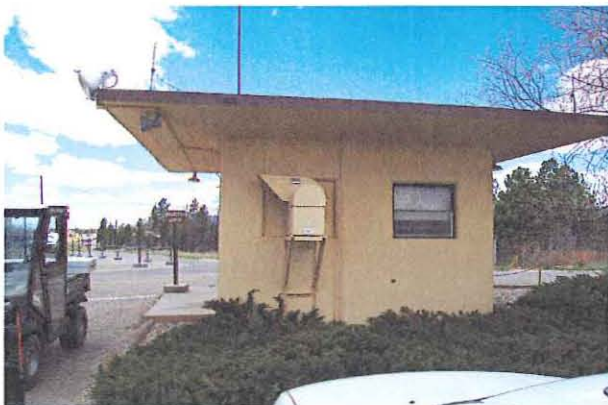
Photo 4c. View of north side of TA-15-46
