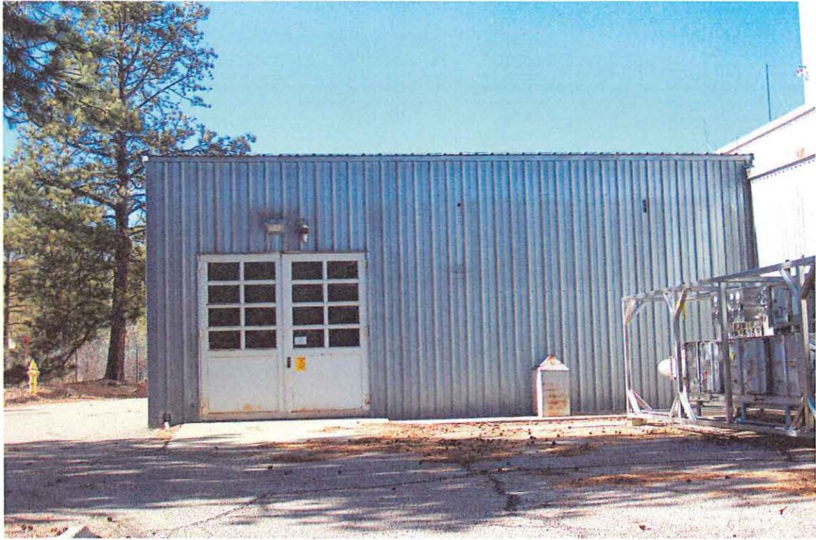
TA-3-16, East elevation, photo 7
