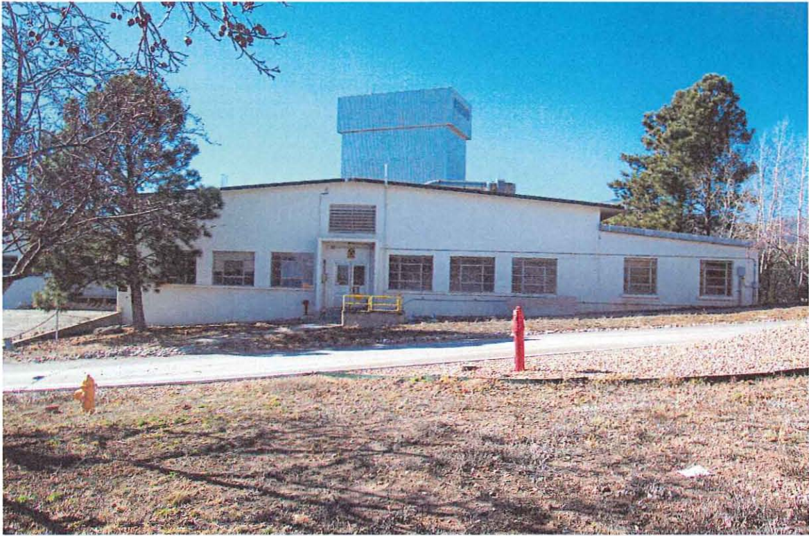
TA-3-16, East elevation, north half, photo 1
