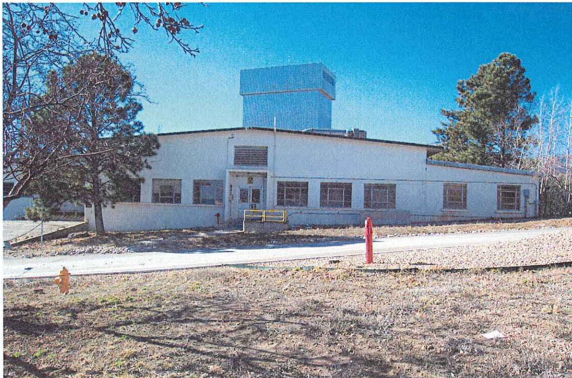
Figure 2. TA-3-16, Front Entrance (office portion)
