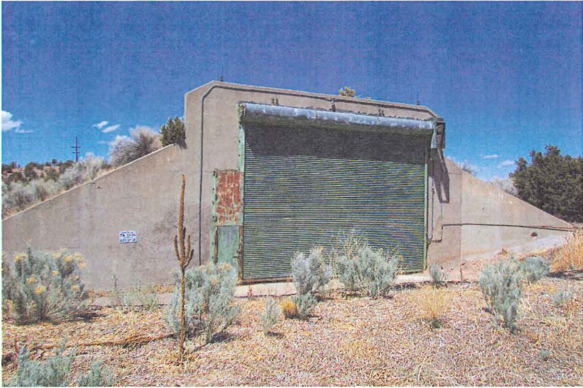
TA-33-25, South side, direction northeast
