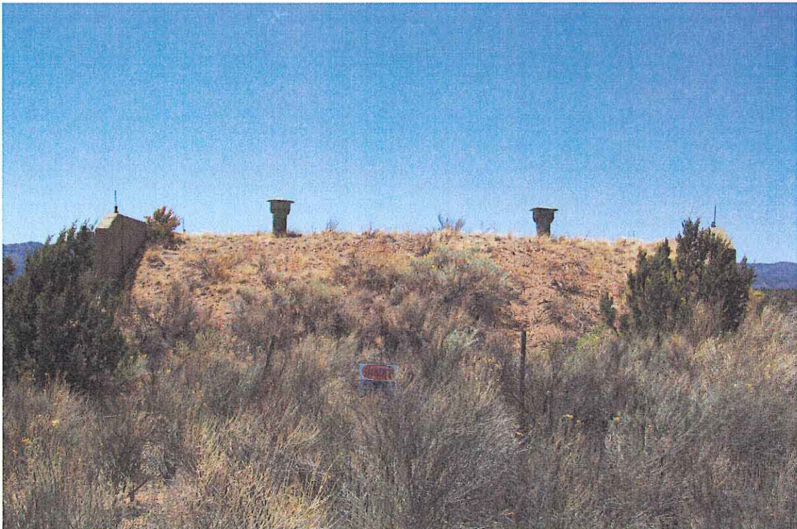
TA-33-25, West side, direction east
