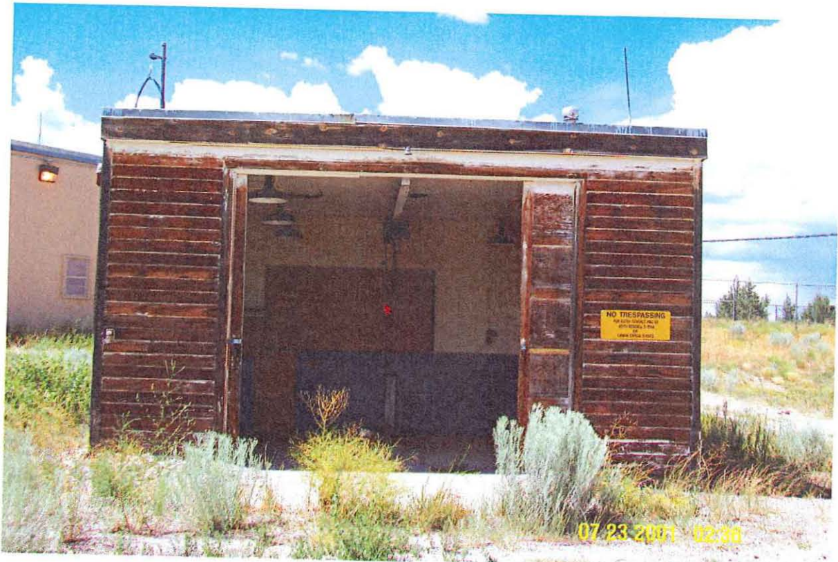
TA-33-40 South Elevation and Interior
