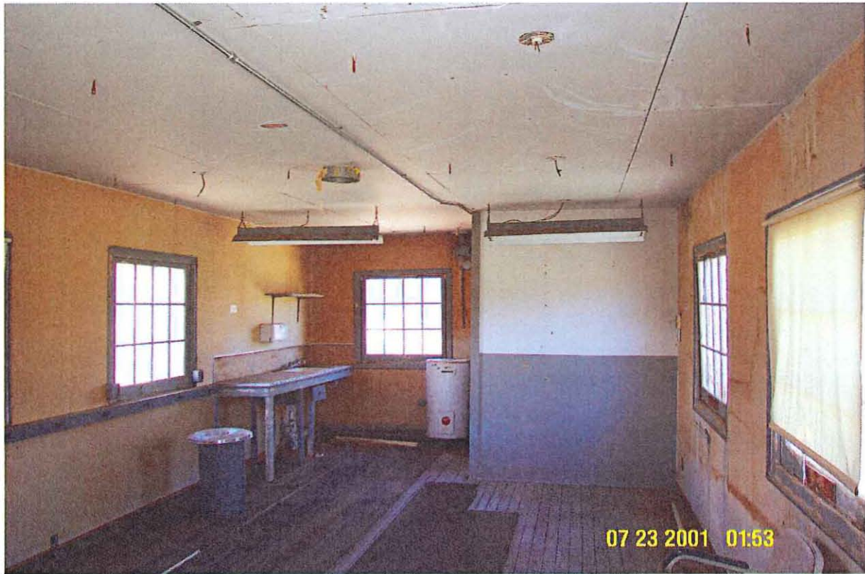
TA-33-1 Interior looking East
