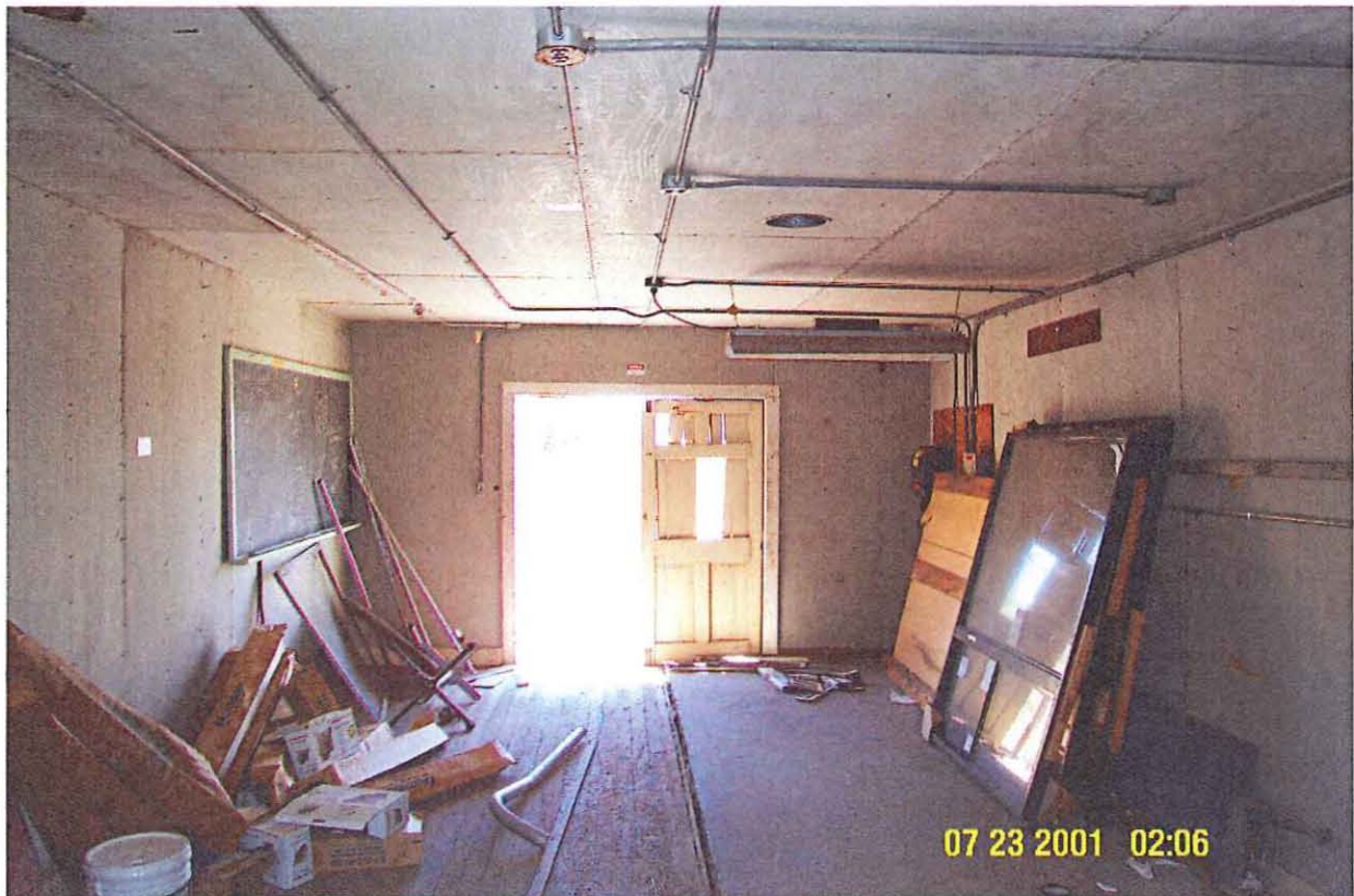
TA-33-2 Interior looking West
