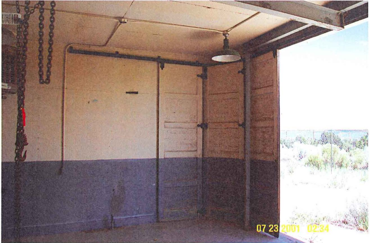
TA-33-40 Interior Sliding Section Door looking southeast
