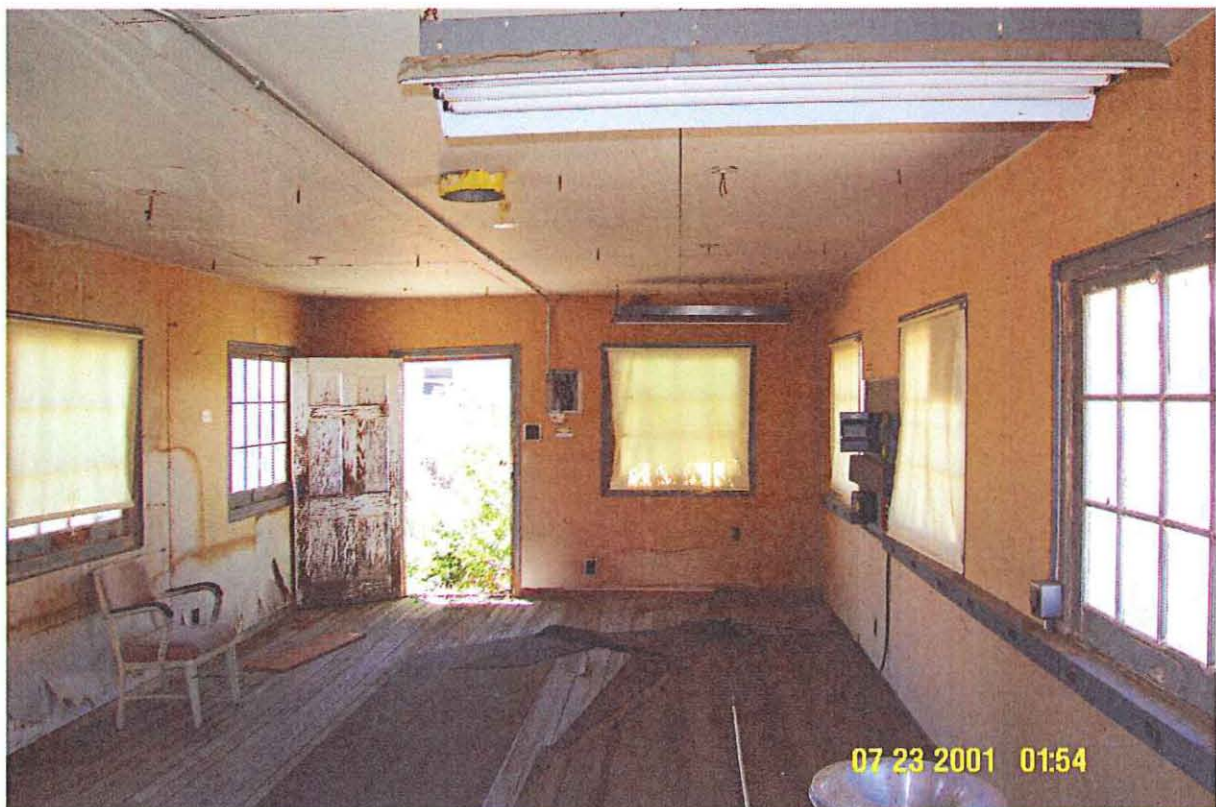
TA-33-1 Interior looking West
