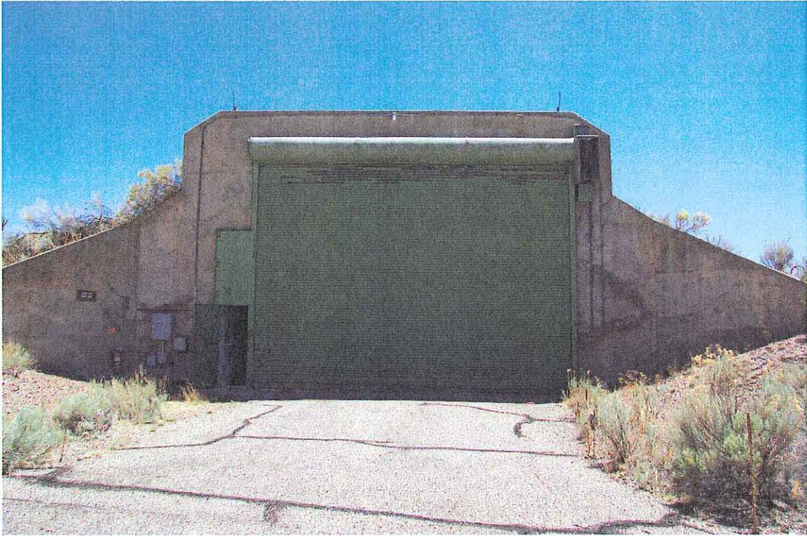
TA-33-25, North side, direction south
