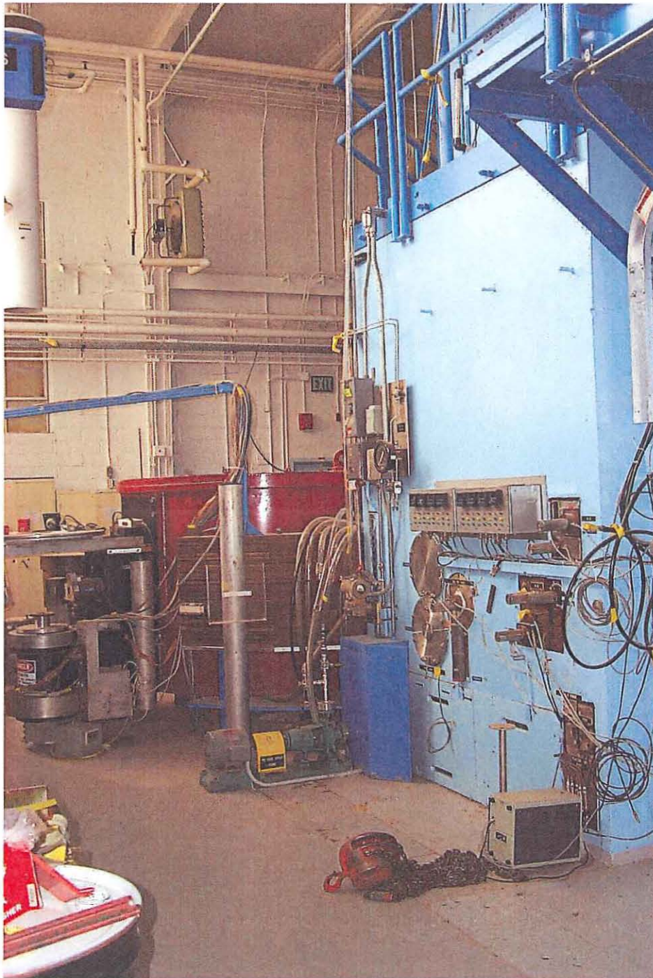
TA-2-1, Omega West Reactor, room 101, south side
