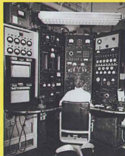
SUPO "Water Boiler" Control Panel
