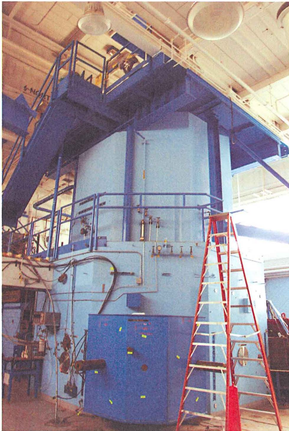
TA-2-1, Omega West Reactor, room 101, north and northwest sides
