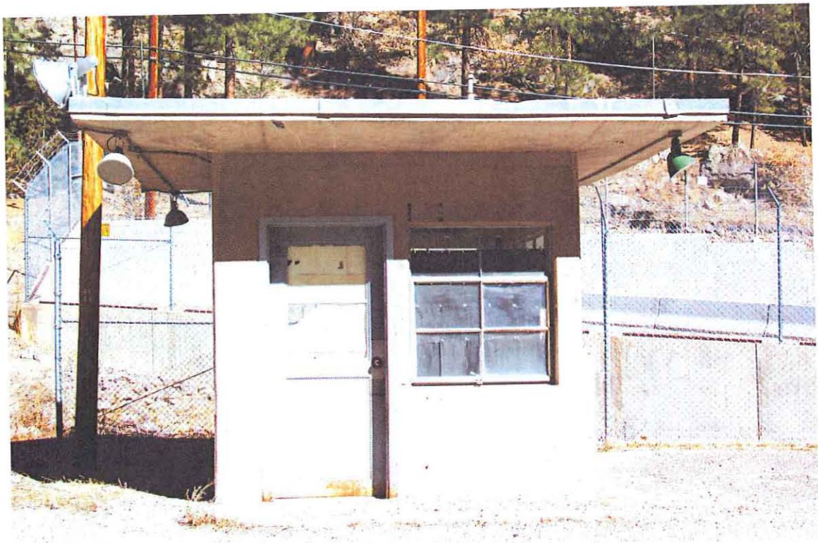
TA-41-16 Guard Station, South Elevation
