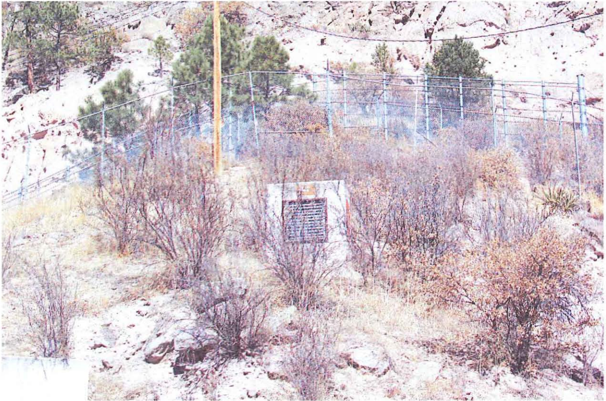
TA-41-3 Blower House Air Intake, South Elevation
