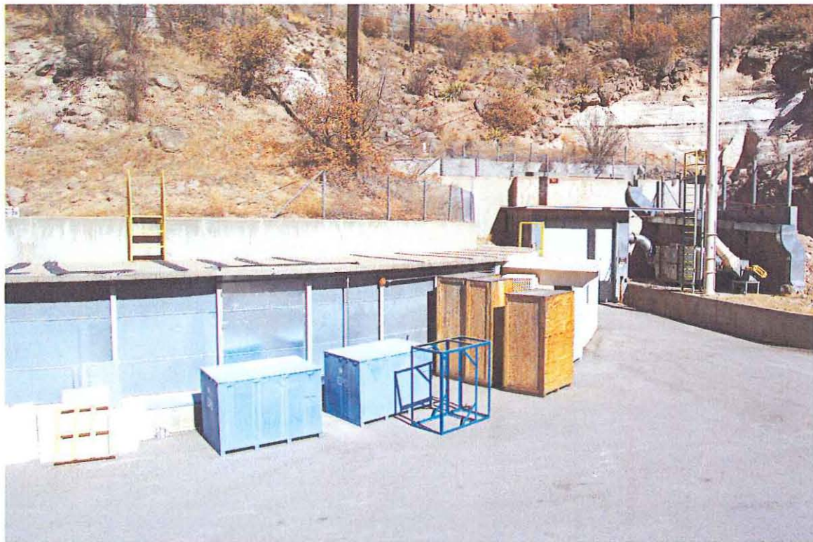
TA-41-6 Passageway, Connecting Building TA-41-1 (on right) to building TA-41-4, South Elevation
