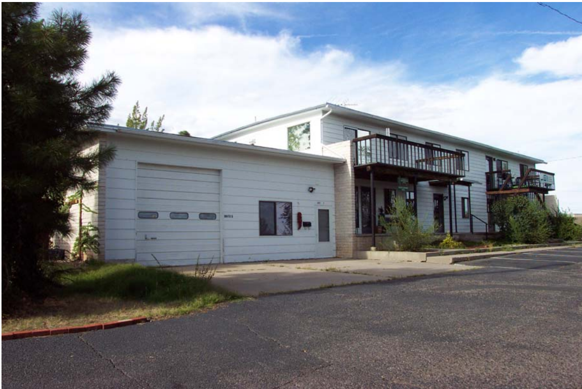
The Last Sundt Building (2 nd Phase Flat Roof Quadruplex), Former Manhattan Project Housing (built circa 1943), Direction North
