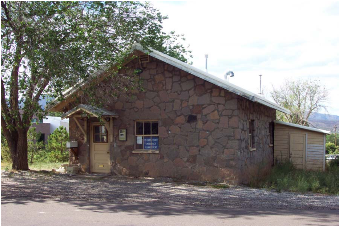
The Red Cross Building, Former Los Alamos Ranch School Power House and Manhattan Project Residence (built early 1930s), Direction Northwest
