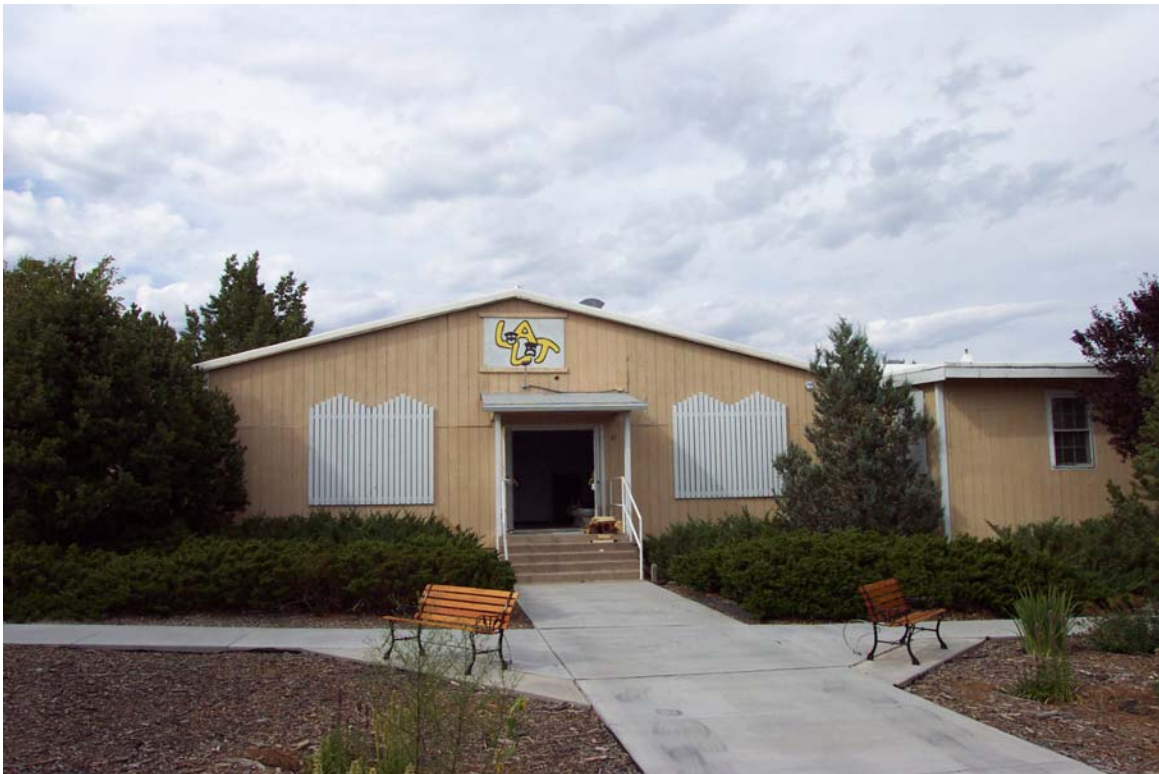
Performing Arts Building, Direction North
