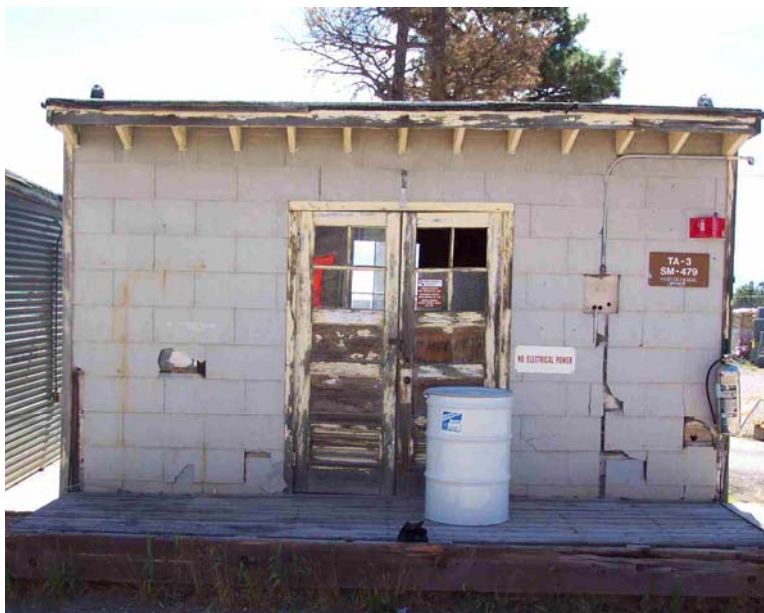
(LANL, RRES-ECO) Manhattan Project Era Building, TA-3
