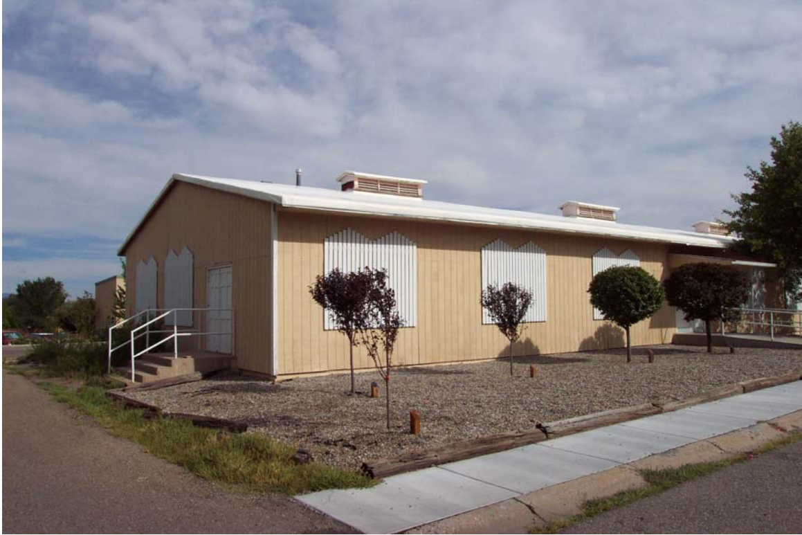
Performing Arts Building, Former Manhattan Project “East Cafeteria” then “Rec Hall” (built early 1940s), Direction Southeast
