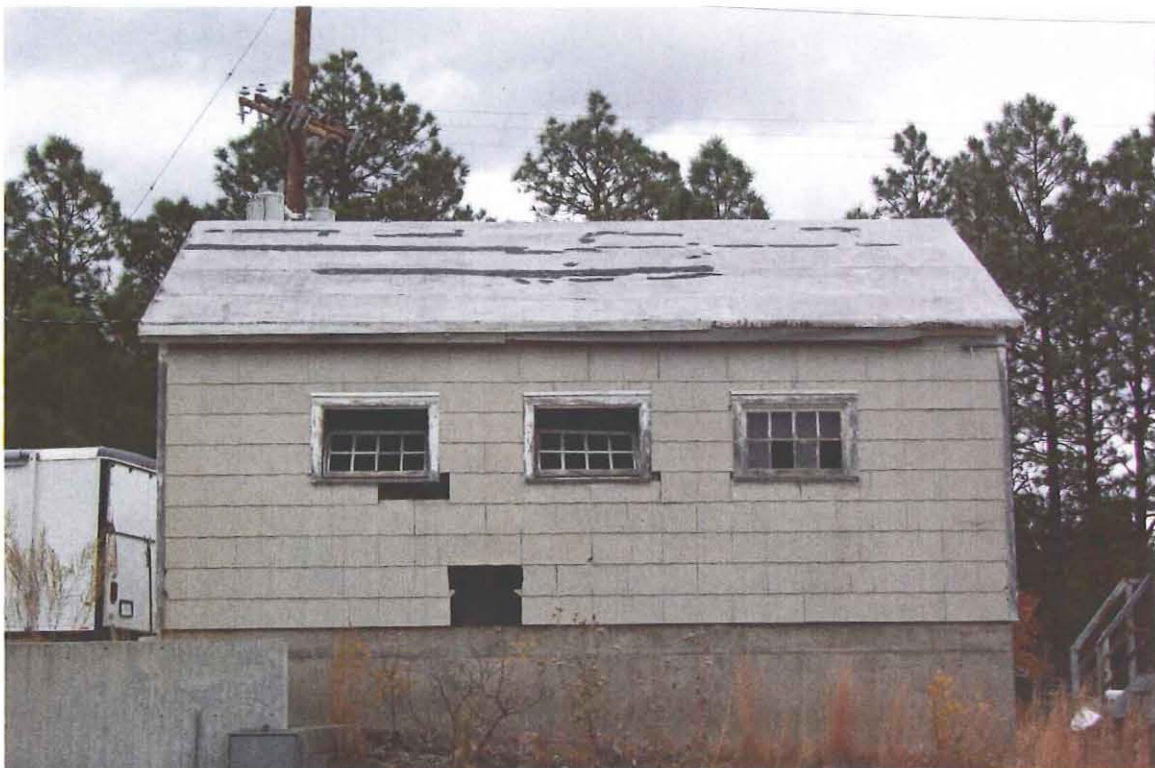
Basket Washing Building, TA-16-390, West Elevation
