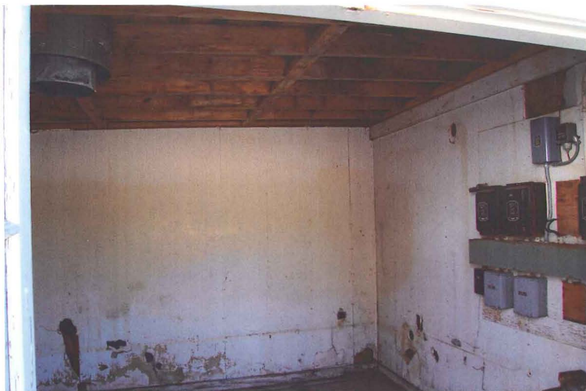
Basket Washing Building, TA-16-390, Mechanical Room Interior, Direction Southwest
