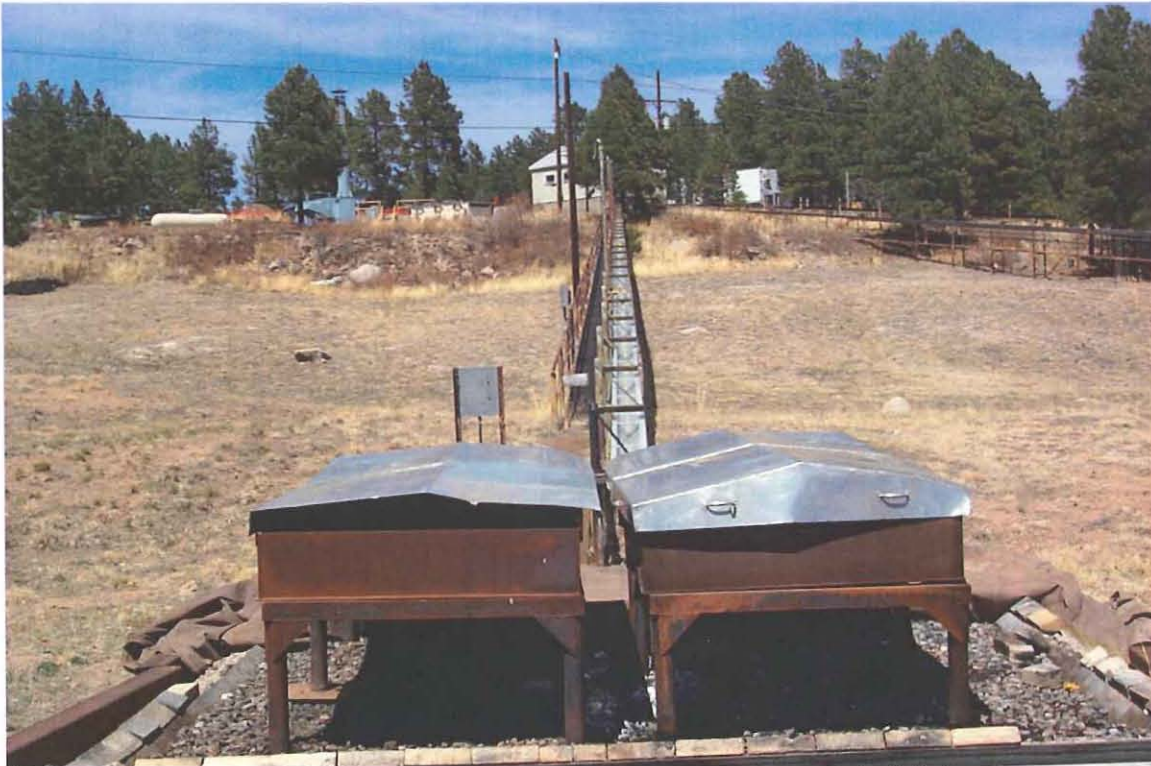
Solvent Burning Trays TA-16-394 (before removal) and Trough TA-16-1134, Direction North
