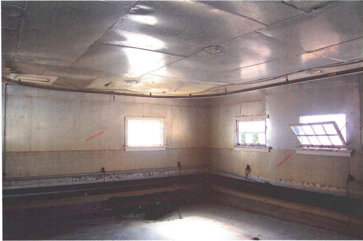
Basket Washing Building, TA-16-390, Interior, Direction Southwest
