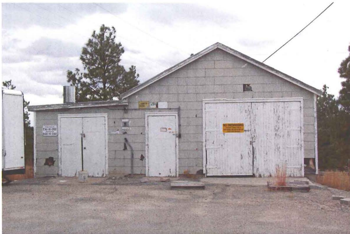
Basket Washing Building, TA-16-390, North Elevation
