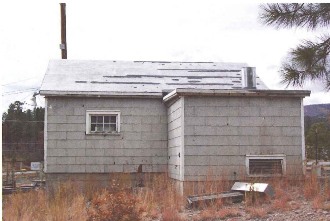
Basket Washing Building, TA-16-390, East Elevation
