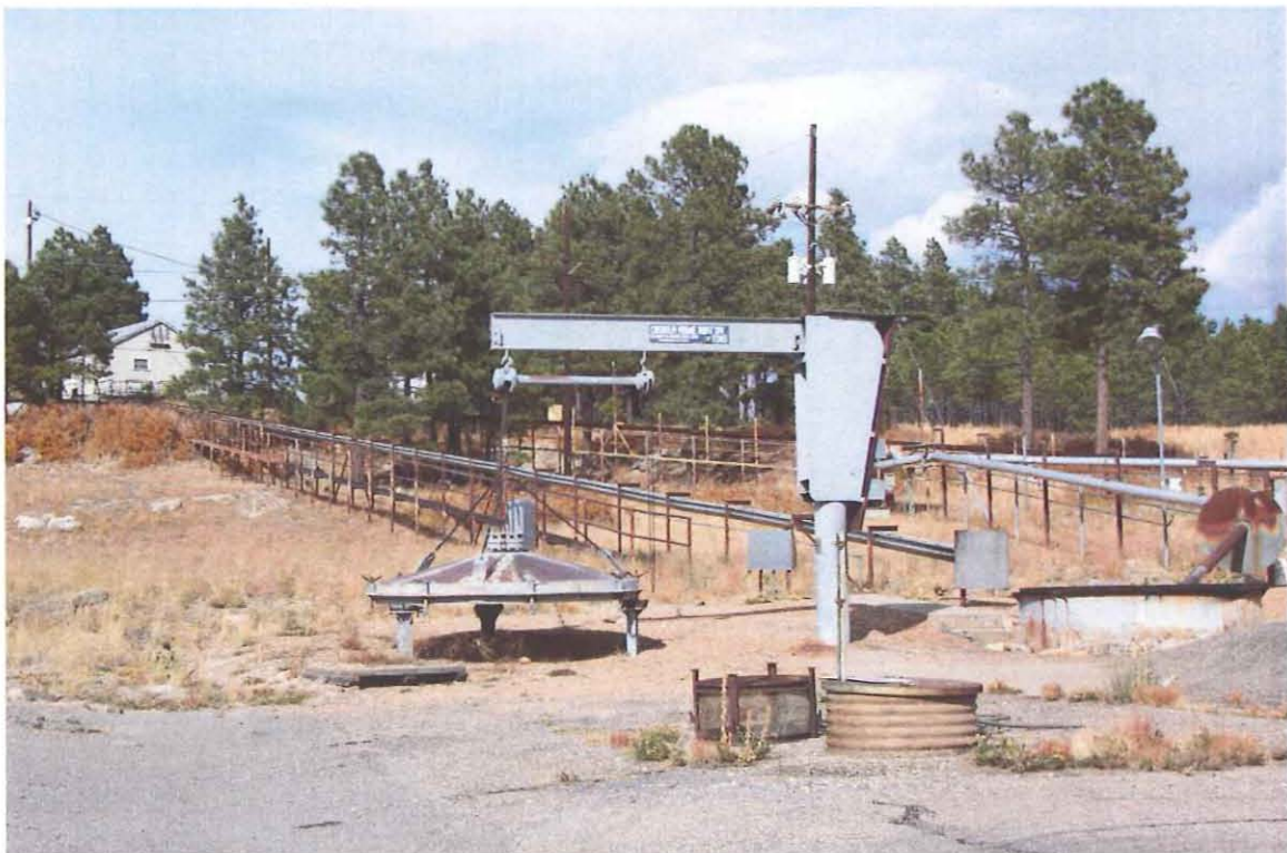
Trough TA-16-1129 and Filtration Vessel and Lid TA-16-401, Direction Northeast
