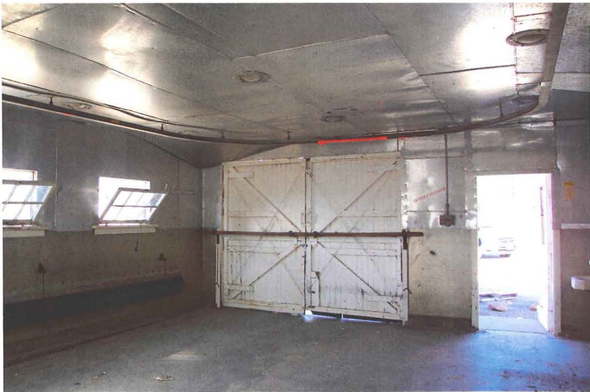
Basket Washing Building, TA-16-390, Interior, Direction Northwest
