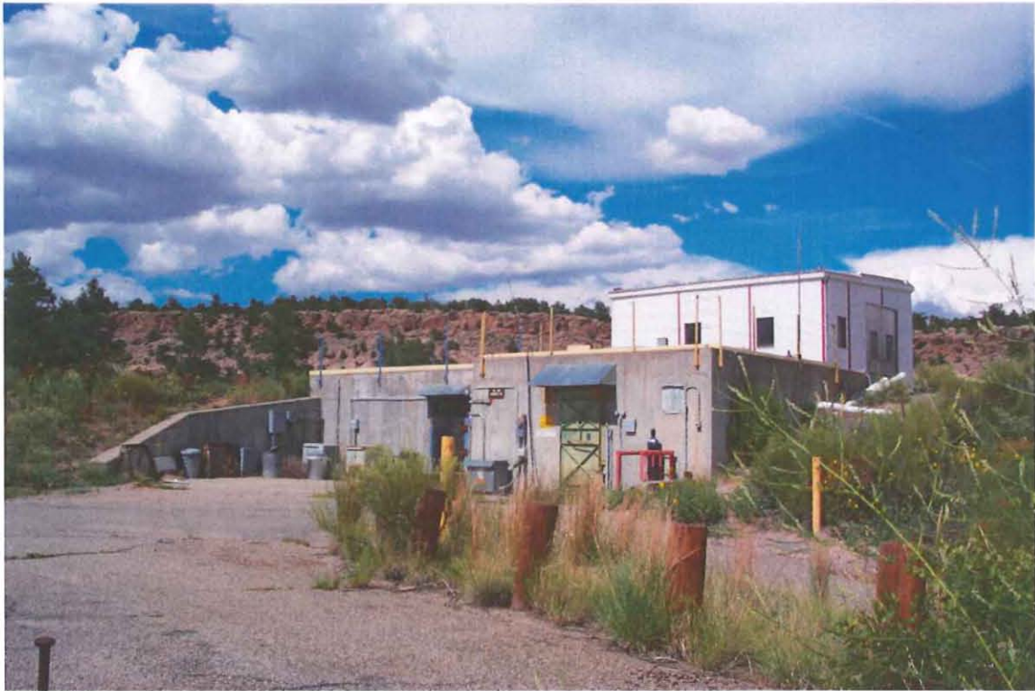
TA-36-12 West and South Elevations. White metal building, TA-15-376 in background.
